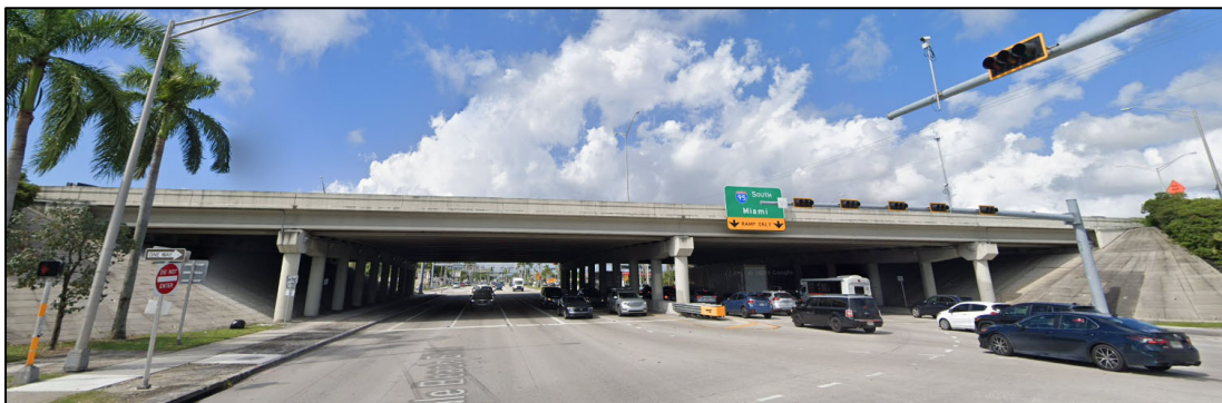
Figure 4.18 - Bridge 860529 - I-95 NB Over Hallandale Beach Blvd.
