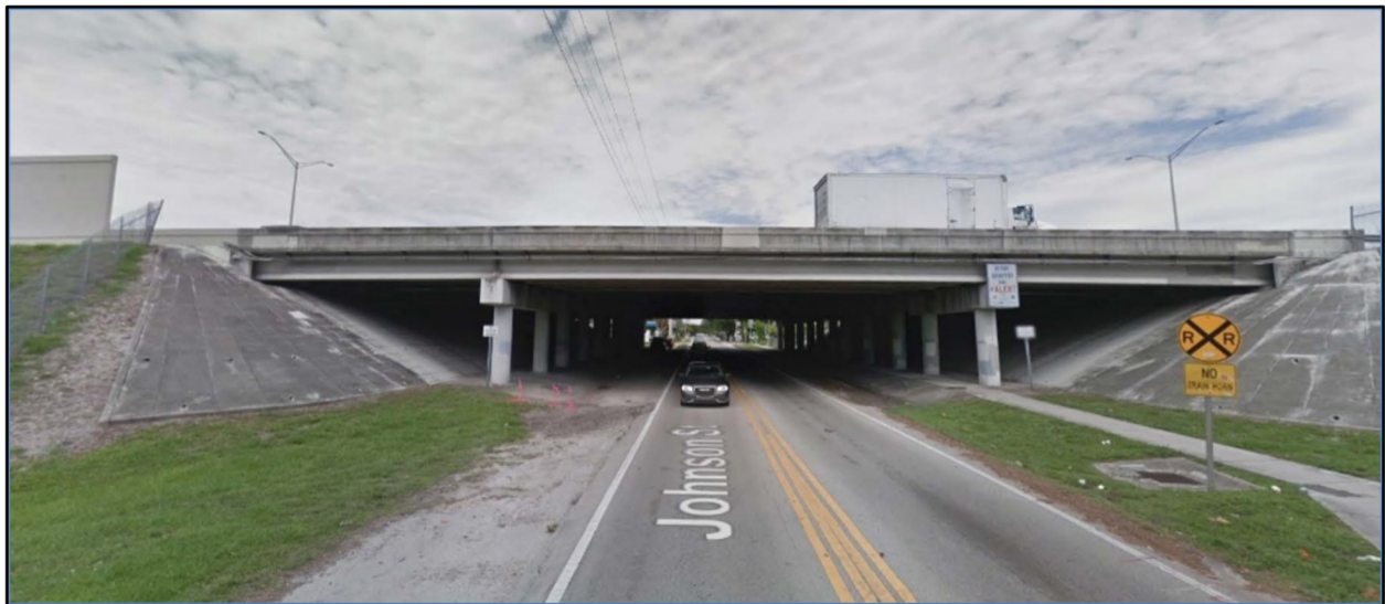
Figure 4.17 - Bridge 860202 - I-95 NB Over Johnson Street
