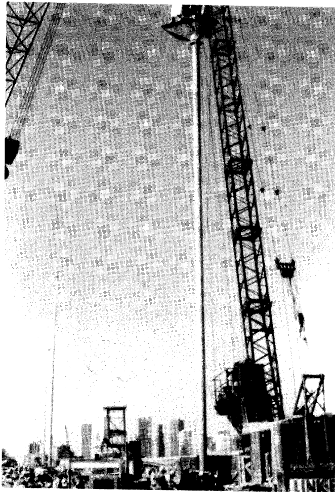
Figure 8.11. Photograph of gravity-fed tremie partially extracted
