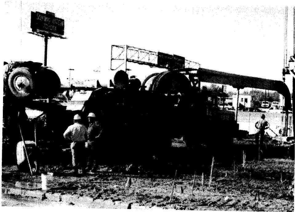
Figure 8.17 a. Pumping operation with a portable, "tremieless" pump unit that does not require a crane to hold the pump line
