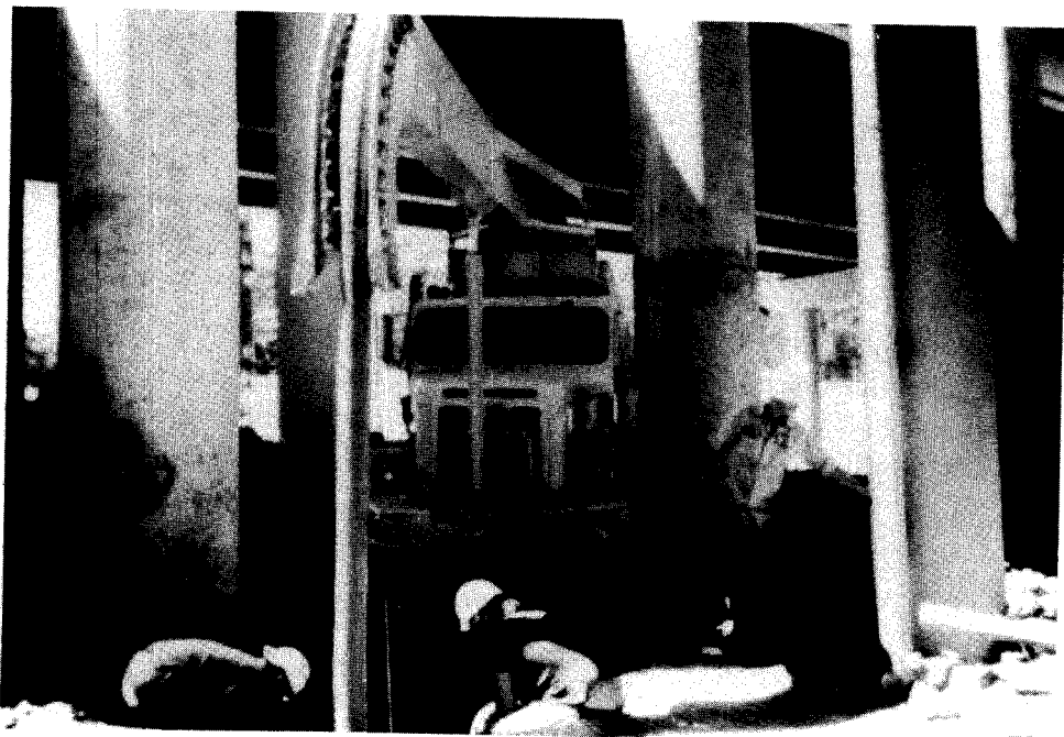
Figure 8.17 a. Pumping operation with a portable, "tremieless" pump unit that does not require a crane to hold the pump line
