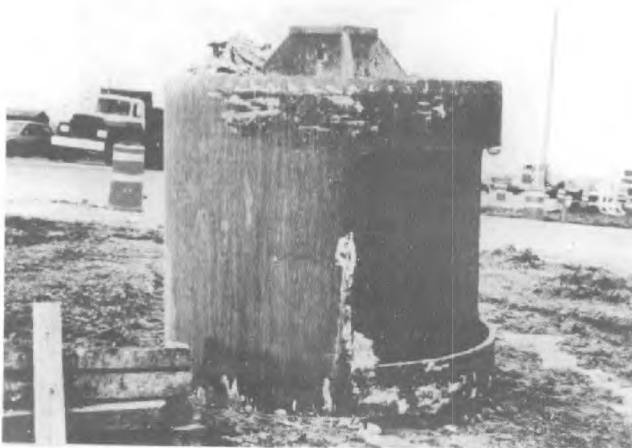
Figure 4.6. A typical "muck bucket" or "clean-out bucket"
