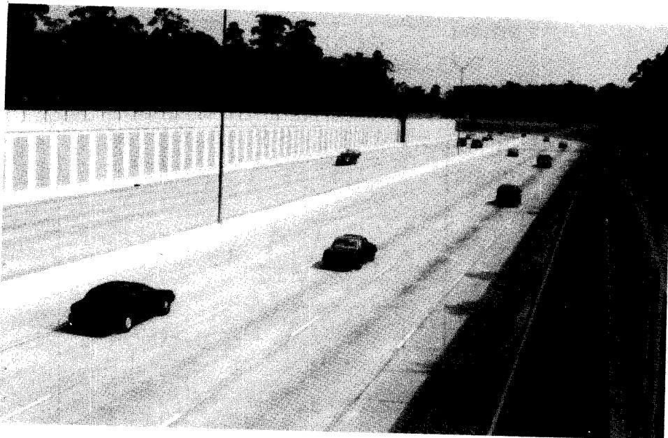
Figure 13.11. Drilled shaft retaining structure for depressed section of highway
