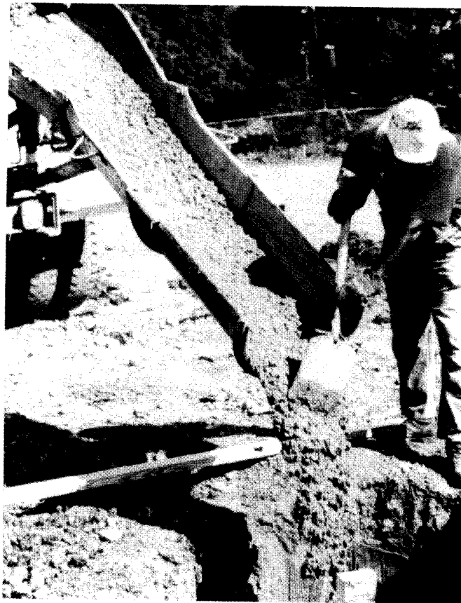
Figure 8.5. Placing concrete directly from the ready-mix truck without a dropchute
