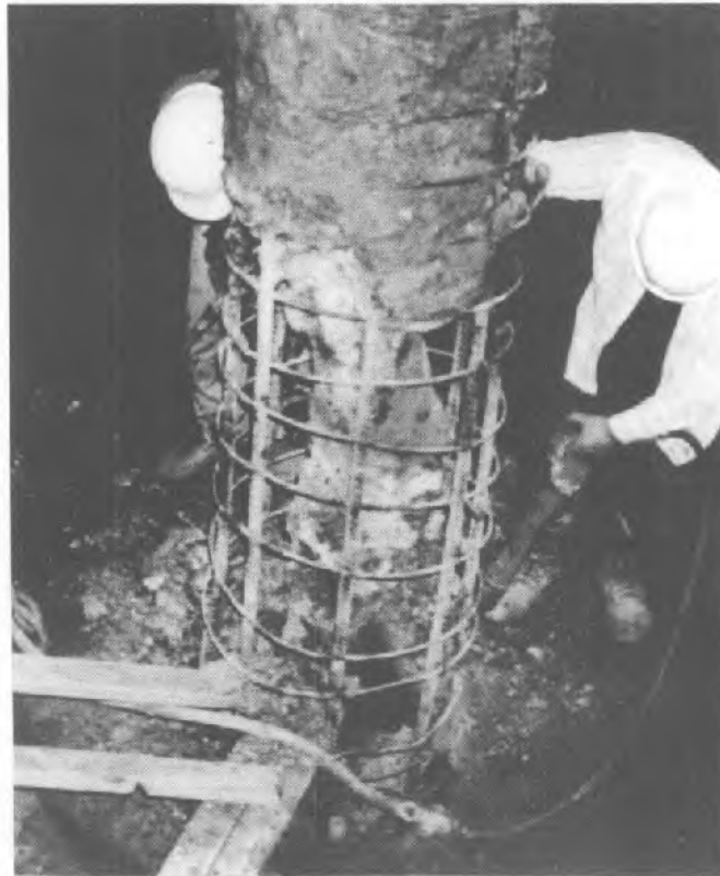
Figure 17.2. A severe defect that can likely be detected by sonic echo testing
