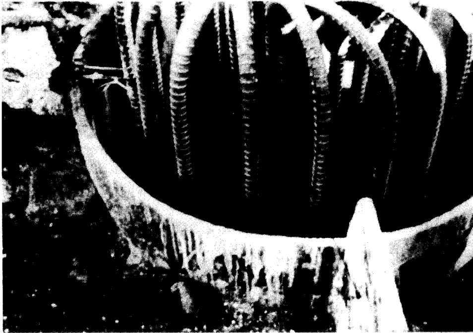
Figure 7.14. Inward-turned hooks in a rebar cage for a drilled shaft at an abutment (photograph courtesy of Barry Berkovitz, FHWA)
