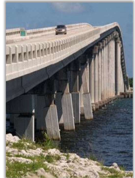
Card Sound Road Bridge – Monroe County SCOP Project District 6
