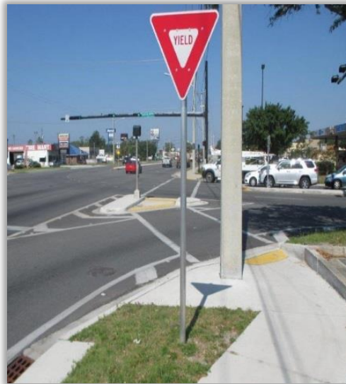
Traffic Operations Improvement, Columbia County CIGP Project, District 2
