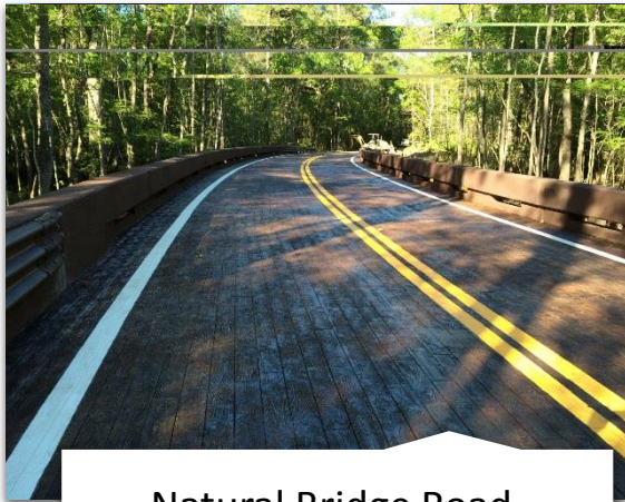
Natural Bridge Road, Leon County
