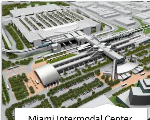
Miami Intermodal Center, Miami Dade County TRIP Project
