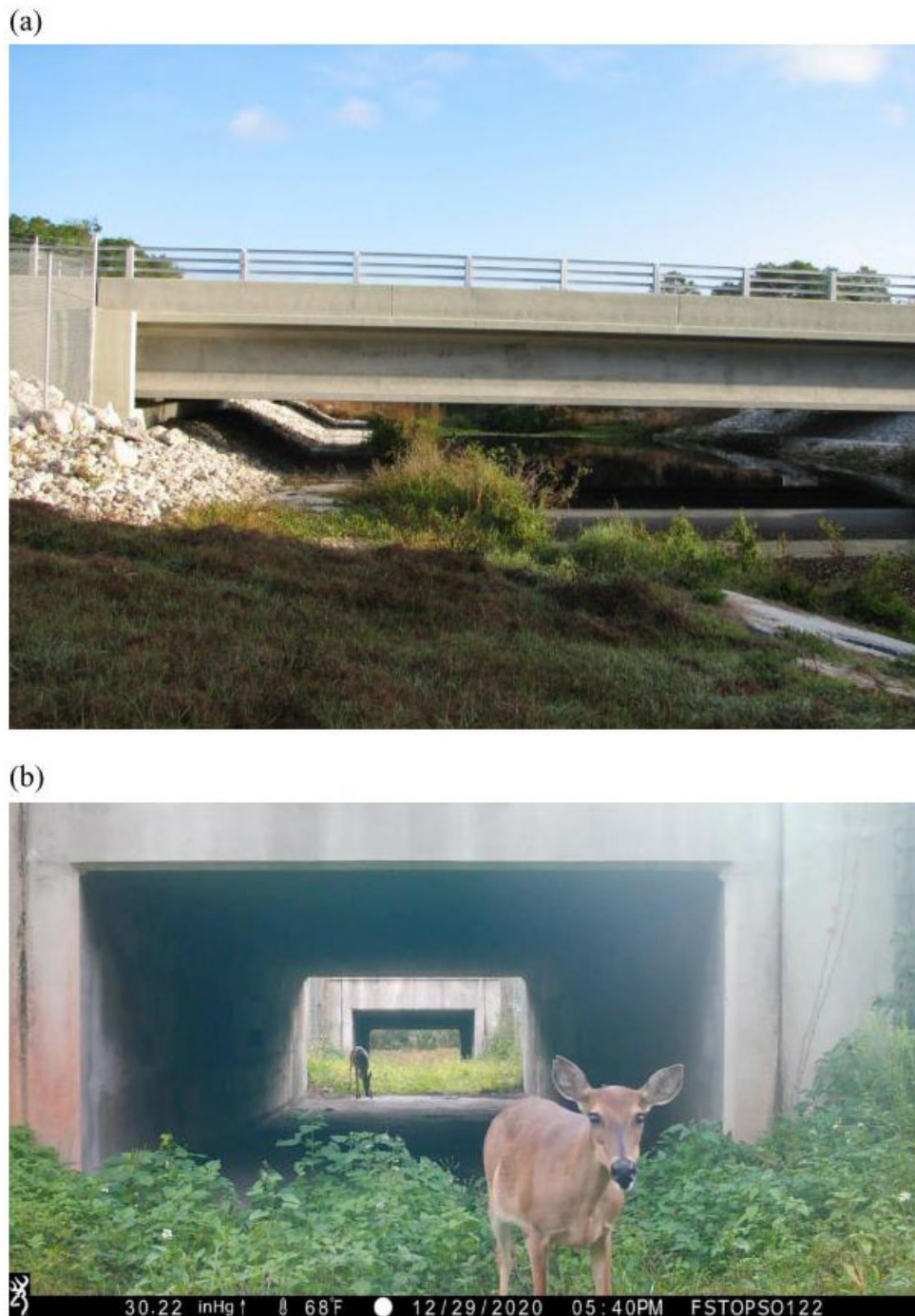
FIGURE 2 Images of wildlife crossings similar to those proposed on State Road 40. (a) A pair of 2.43-m-wide shelves under State Road 80 near the C-1 Canal, east of LaBelle, Florida. Photo credit: Florida Department of Transportation. (b) A 3.04-m-wide \times 1.67-m-high concrete box culvert under State Road 60 at Padgett Branch, near Fort Drum Wildlife Management Area. Photo credit: fStop Foundation.
