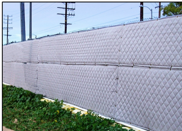
PHOTO 17 – Sound blanket fences ( below ) are an option to help control noise and provide a visual and light barrier.
