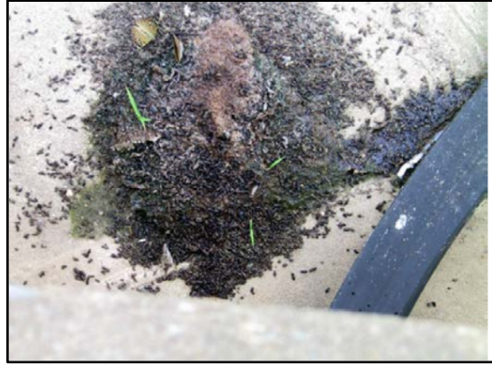
PHOTO 9 - (TOP LEFT) Guano deposit on pier. PHOTO 10 - (TOP RIGHT) Guano from bridge deck, on top of pier.
