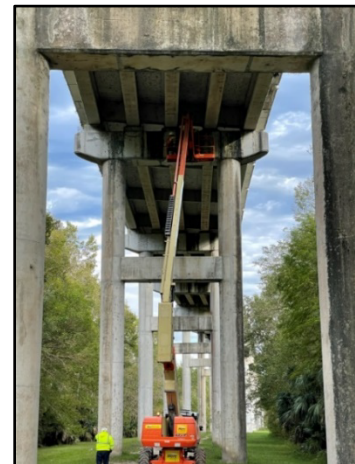
PHOTO 21 - Access Issue - High bridge structures (Ocklawaha River Bridge).
