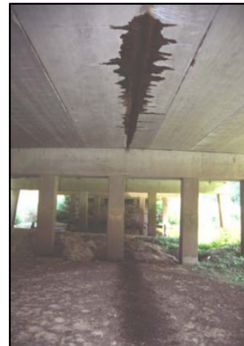
PHOTO 7 - (TOP LEFT) Staining on I-95 Bridge in Fort Pierce. Photo by FWC. PHOTO 8- (TOP RIGHT) Staining along longitudinal joint and guano on ground.
