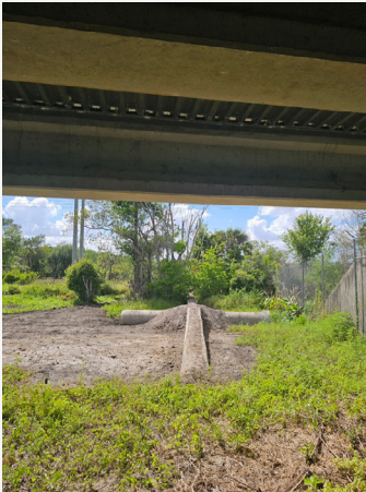
Wooden pile bridge walkway added to SR 29 Pistol Pond Crossing.
