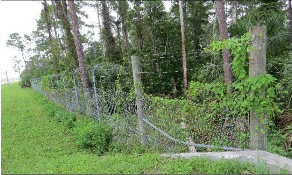
Figure 60 Concrete barrier wall and wildlife fence for a jump out, I-4, Volusia County, D5 (FPID 408464-1).
