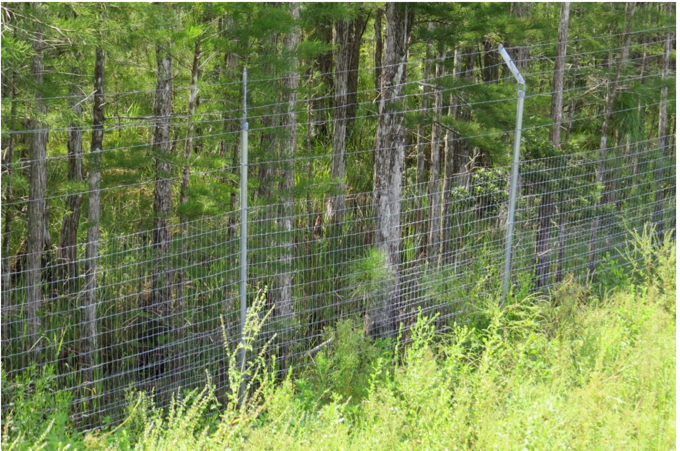
Figure 50 Wildlife fence with woven wire and barbed wire (Type A) on I-4, Volusia County, D5 (FPID 408464-1).
