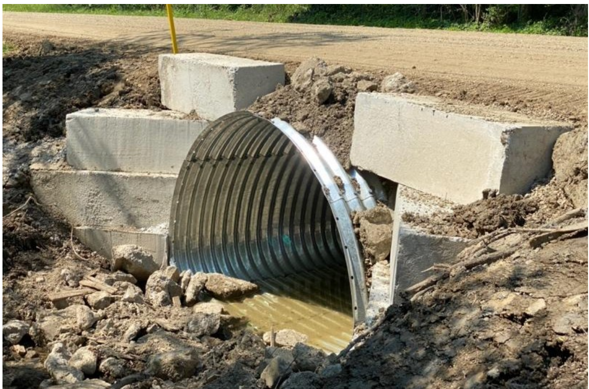
Figure 28 Corrugated steel pipe culvert.
