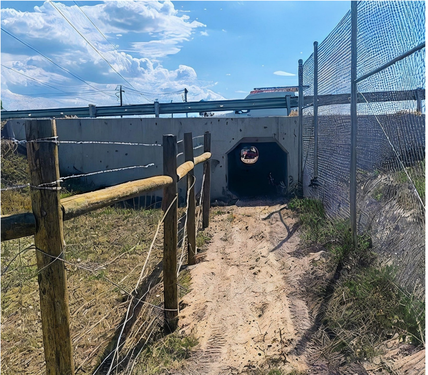
Figure 20 Dry box culvert under SR 55, Polk County, D1 (FPID 201215-3).
