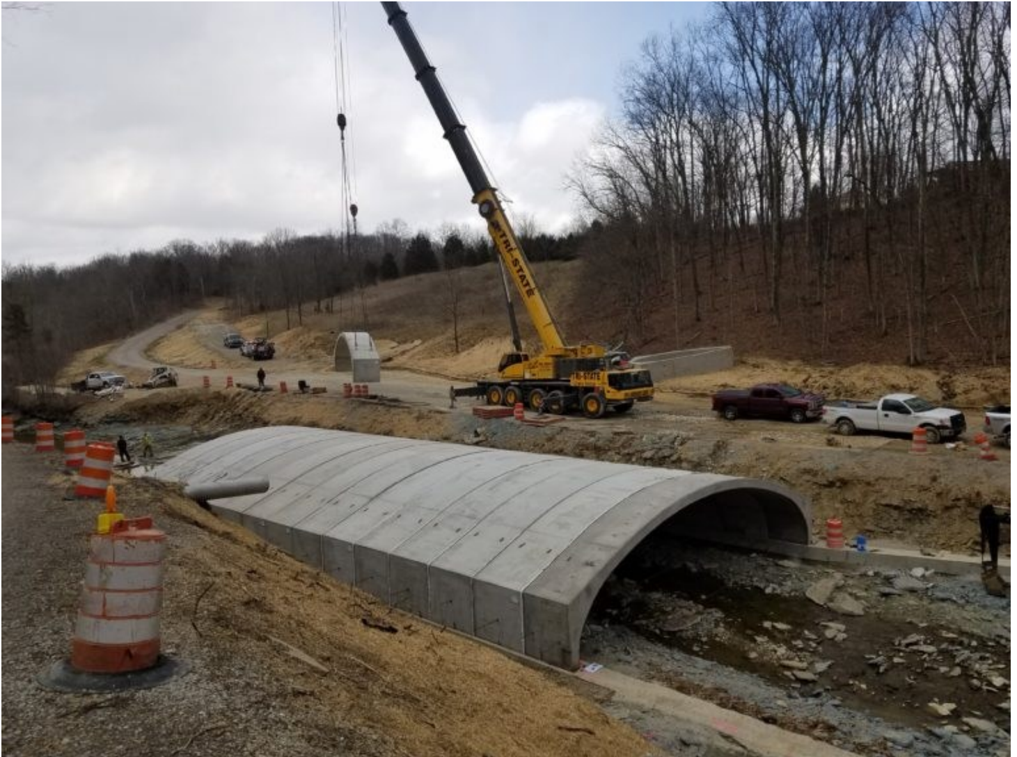
Figure 26 Bridge-sized three-sided concrete culvert.
