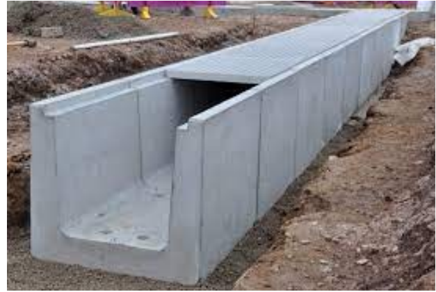
Figure 42 Concrete Vaults that carry Utilities.
