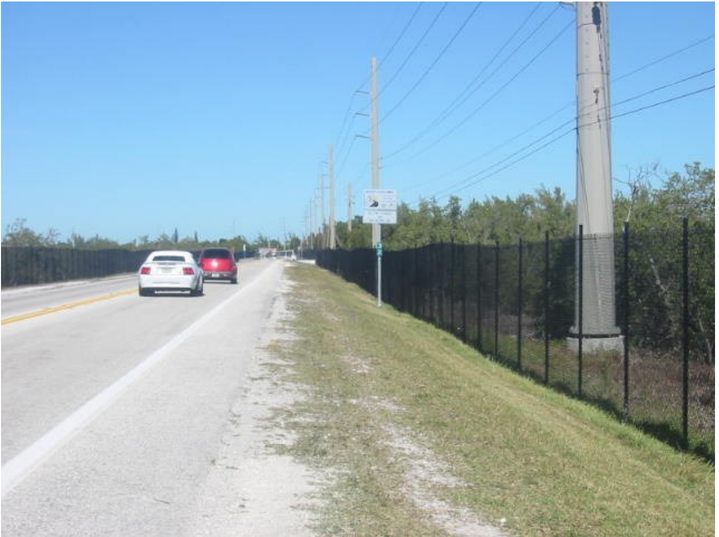
Figure 51 Wildlife fence specifically for key deer on US 1, Monroe County, D6 (FPID 434684-1, 443897-1, and 250564-2).
