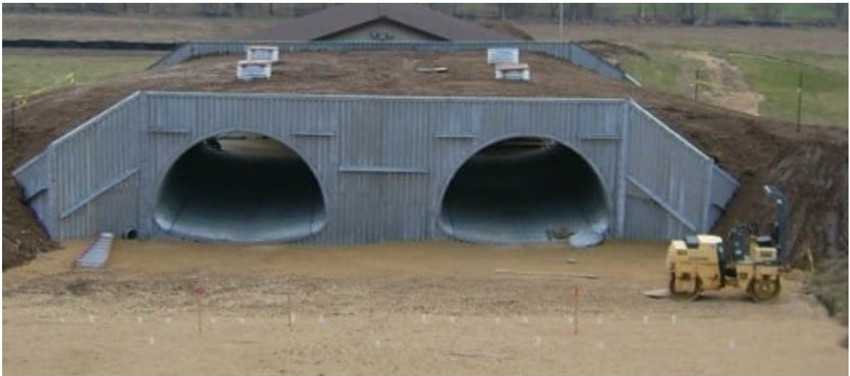
Figure 27 Aluminum Arch-Pipe Culverts
