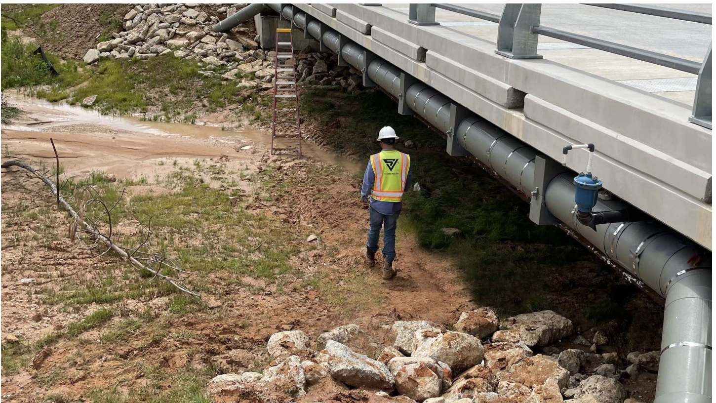
Figure 43 Under-bridge Pipe Addition.
