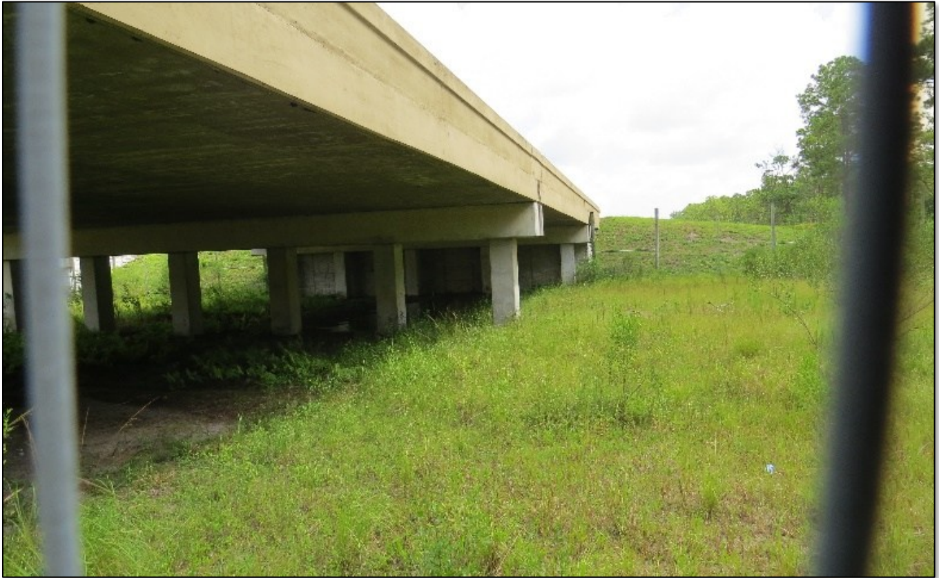
Figure 7 Bridge for dry crossing under I-4 in Volusia County, D5 (FPID 408464-1).
