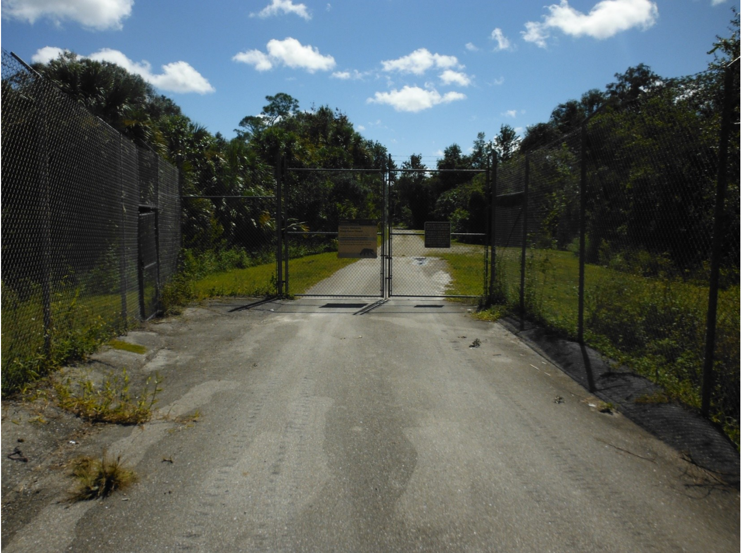
Figure 56 Access gate and swing gate for maintenance within a segment of wildlife fence on SR 29, Collier County, D1 (FPID 407940-1).
