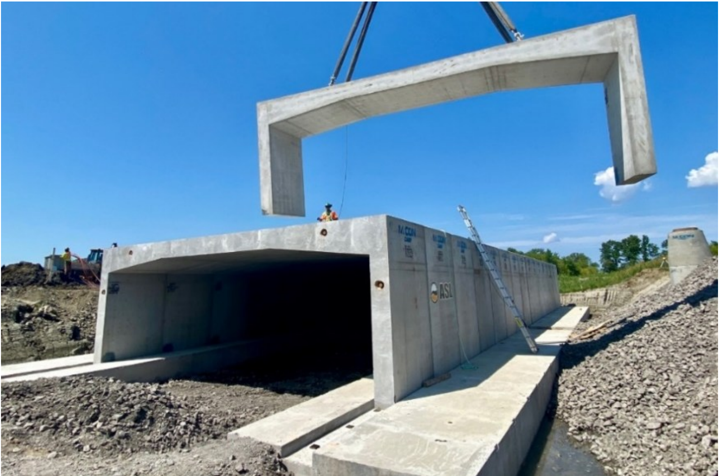
Figure 25 Rectangular three-sided concrete culvert.
