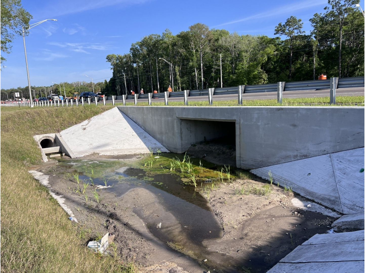
Figure 21 Dry box culvert under SR 52, Pasco County, D7 (FPID 256323-1).
