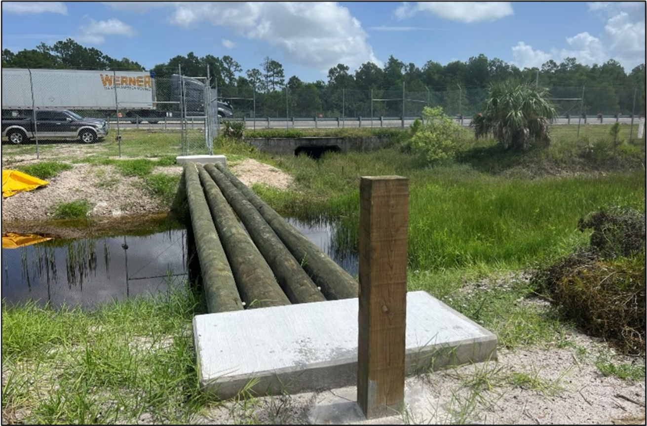
Figure 41 Timber pile bridge, I-75 Alligator Alley, Collier County, D1 (FPID 444008-3).
