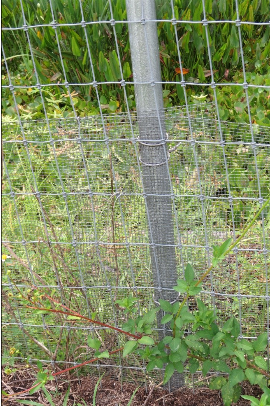
Figure 52 Herpetofauna fence attached to woven wire fence, I-4, Volusia County, D5 (FPID 408464-1).
