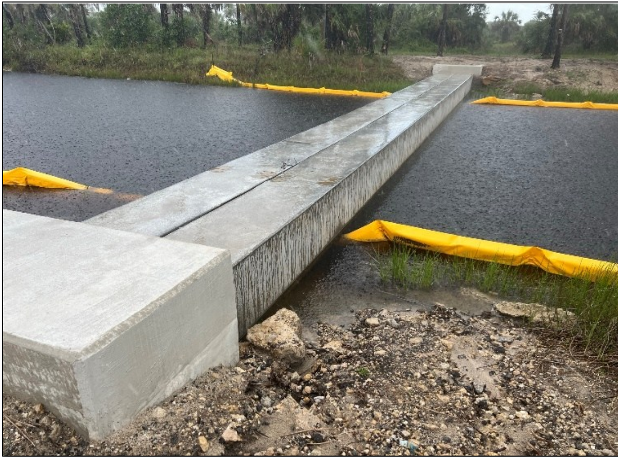
Figure 39 Concrete pile bridge, I-75 Alligator Alley, Collier County, D1 (FPID 444008-3).
