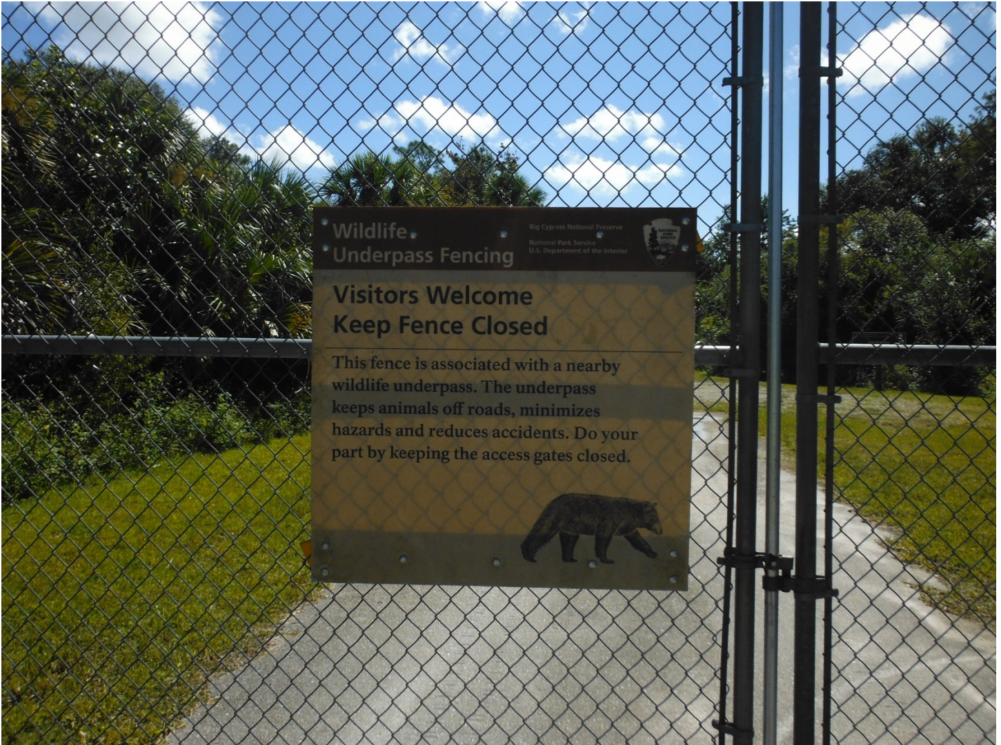
Figure 55 Example of public awareness sign on an access gate within a segment of wildlife fence, SR 29, Collier County, D1 (FPID 407940-1).
