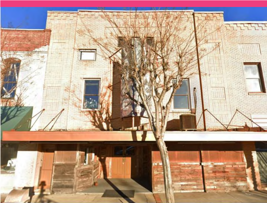
An example of alterations to a pre-war (1901) commercial building at 499 Main Street (Washington County). Alterations include modern windows and cladding on the first floor.
