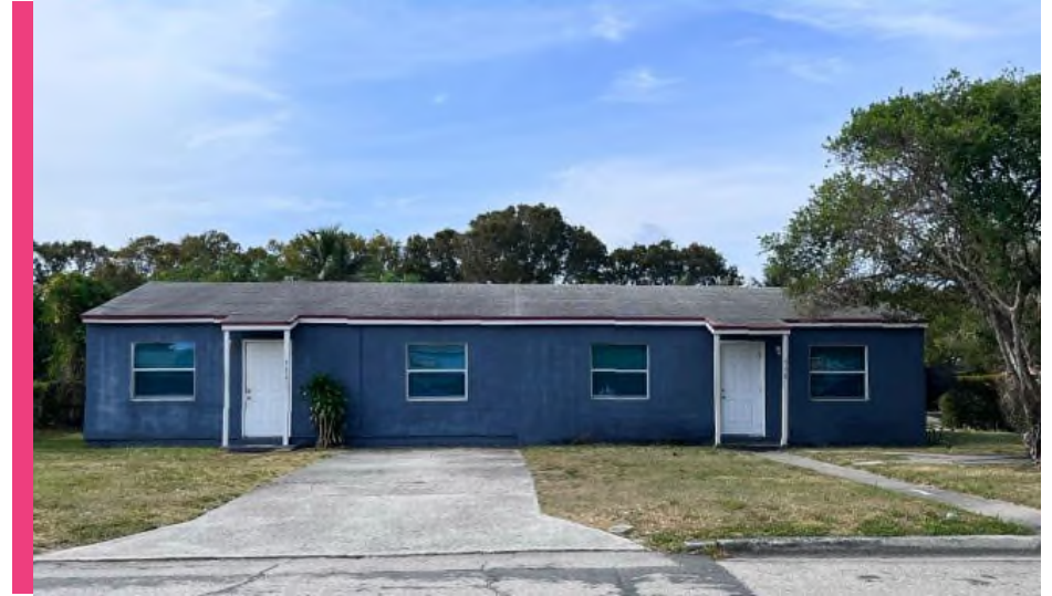
A structure with major alterations at 738 49th Street (Palm Beach County), constructed in 1947. Alterations: new siding, new windows, enclosed garage, addition of new entrance, conversion of structure from single-family residence to multi-family residence
