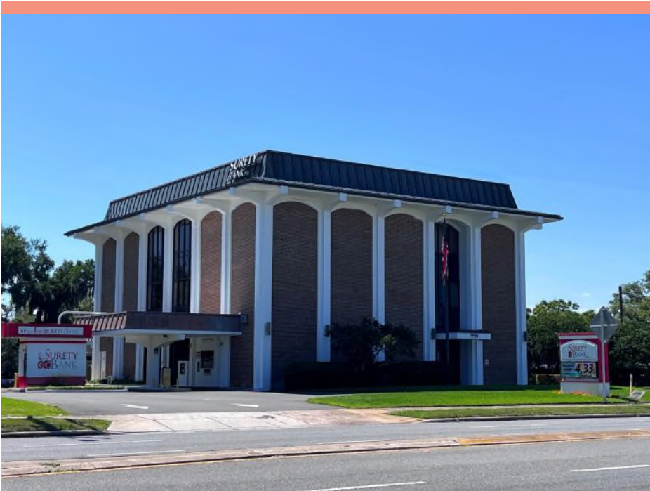
A New Formalism Style commercial building at 990 Woodland Boulevard (Volusia County), constructed in 1975
