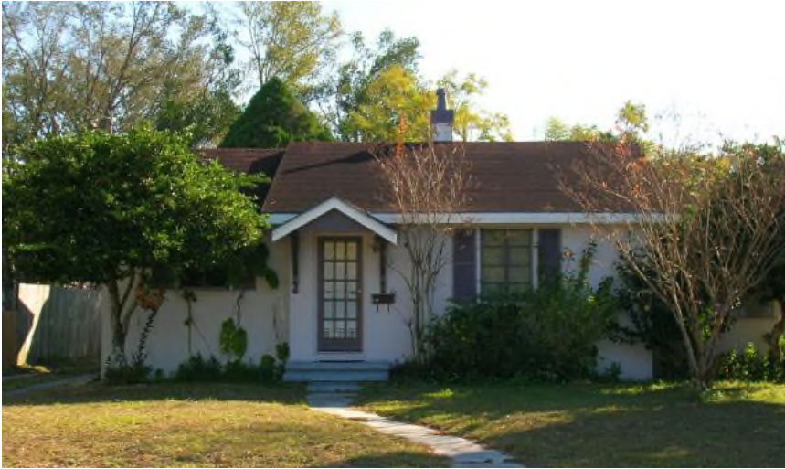
A Masonry Vernacular Style Residence at 104 14th Street SE (Polk County), constructed in 1946 (8PO6919)
