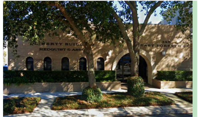
An example of alterations to a post-war (1945) commercial building at 345 E. Forsyth Street (Duval County). Alterations include modern windows and entrance.
