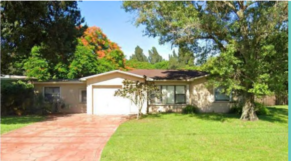
A structure with major alterations at 316 East Acre Drive (Broward County). Alterations: new siding, replacement windows, addition on the front façade (left side)
