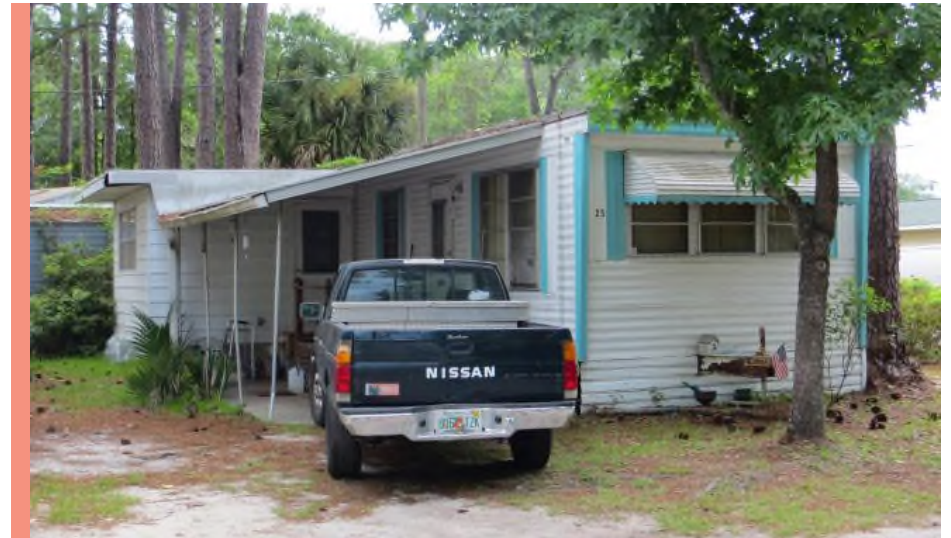
A structure with major alterations at 25 Little Texas Avenue (Bay County). Alterations: new addition (rear left) visible from the front (8BY1834)
