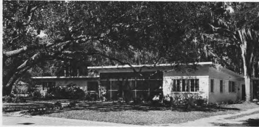
WIDE overhang of semi-flat roof protects interior of Fla. home. Screened-in porch facing street takes advantage of prevailing breezes
