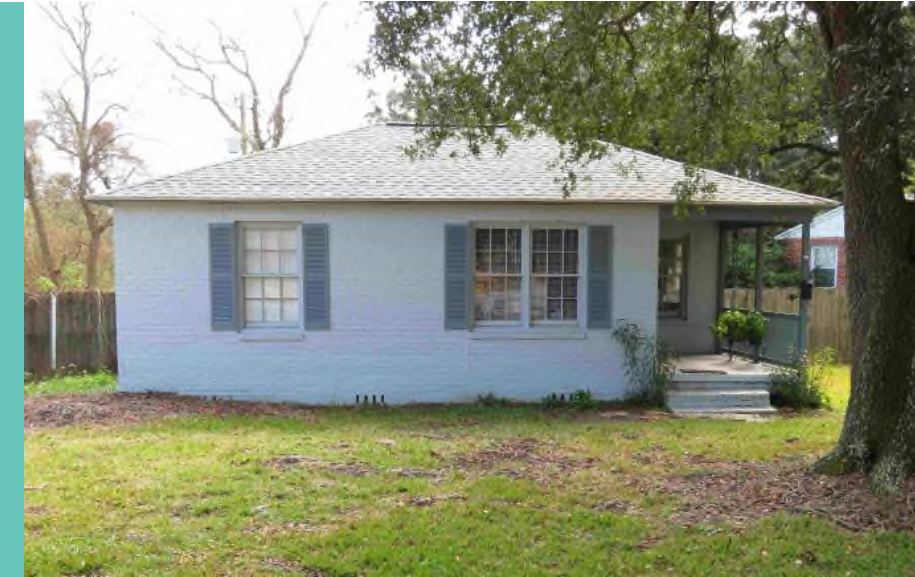
A Bungalow Form Residence at 628 W Sunset Avenue (Escambia County), constructed in 1945 (8ES5207)
