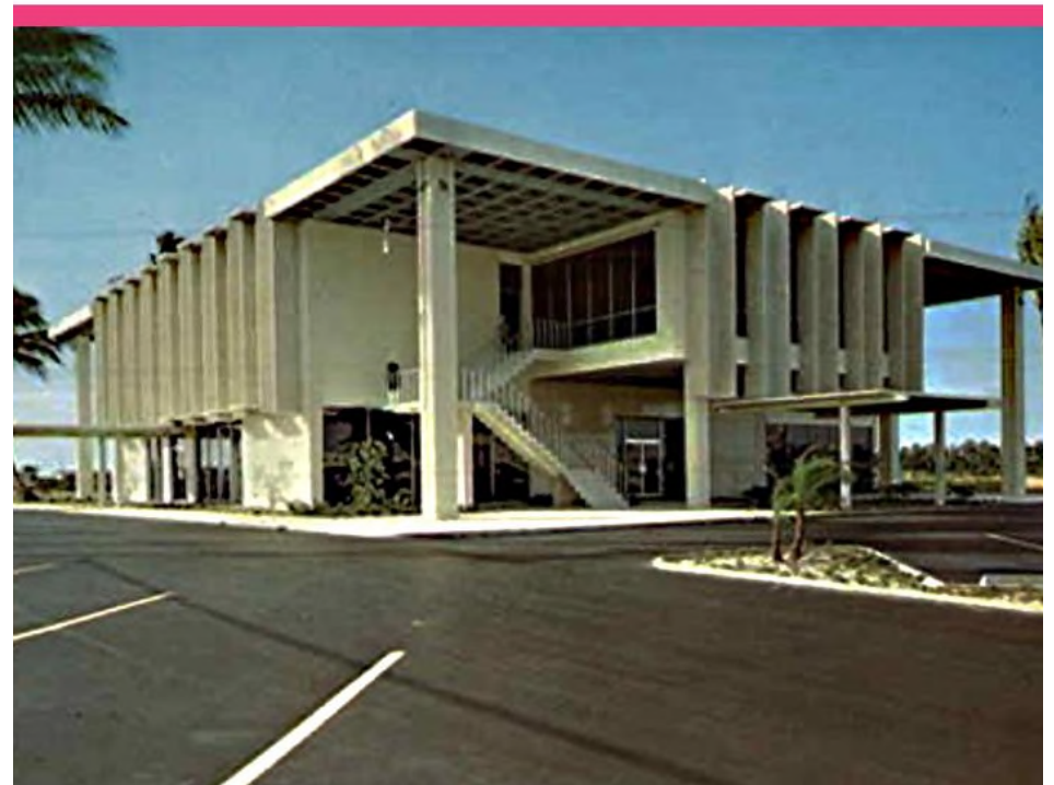
Photograph of First Federal Savings and Loan Association (8PB18601) as it appeared in the 1960s (Photo from post card, accessed from https://www.amazon.com/Federal-Association-Original-Vintage-Postcard/dp/B00P6RFG8I ).
