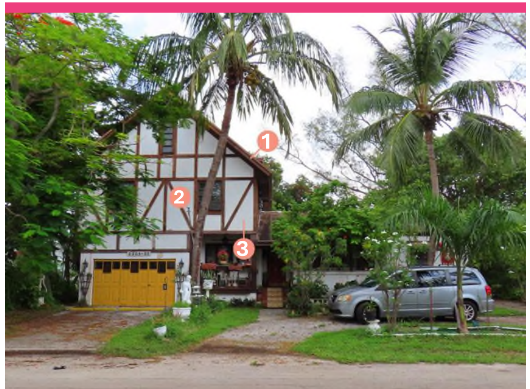
A Tudor Revival Style Residence at 2205-7 Taylor Street (Broward County), constructed in 1950 (8BD9412)
