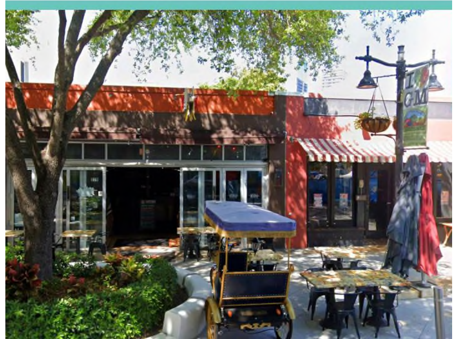
An example of alterations to a pre-war (1929) commercial building at 517-9 Clematis Street (Palm Beach County). Alterations include modern windows and cladding on the first floor.
