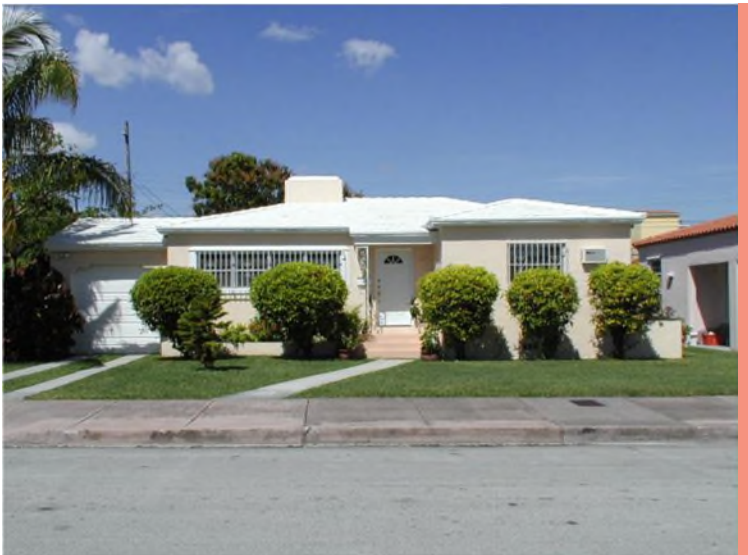
A Minimal Traditional Form Residence at 33 Campina Court (Miami-Dade County), constructed in 1941 (8DA9482)
