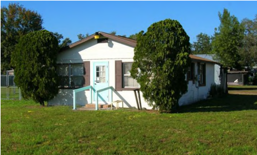
A Masonry Vernacular Style Residence at 2255 State Road 542 (Polk County), constructed in 1953 (8PO6941)
