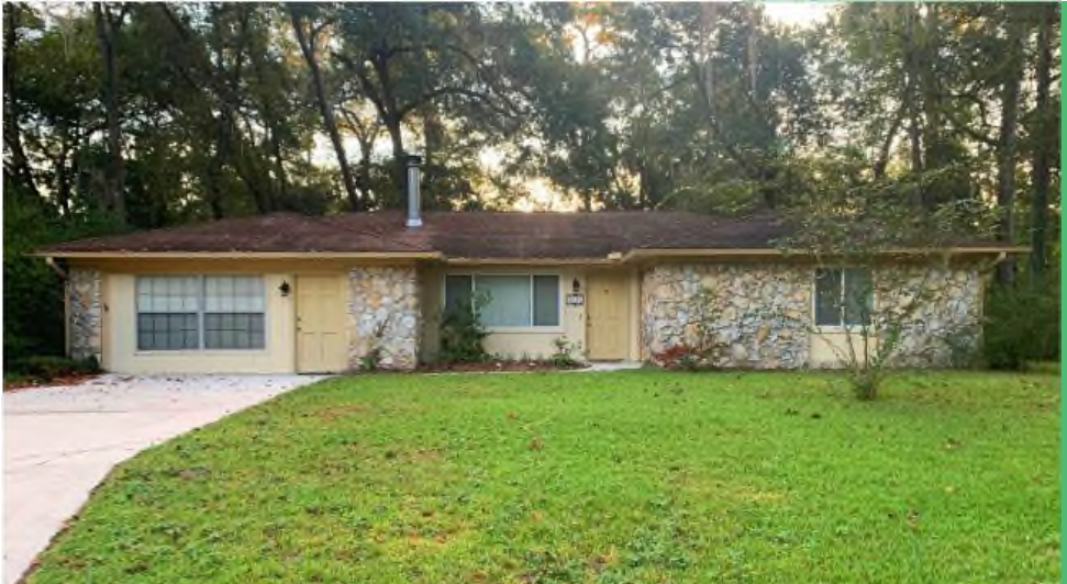
A structure with major alterations at 4617 NW 42nd Street (Alachua County): Alterations: new siding, replacement windows, enclosed garage, new second entrance.
