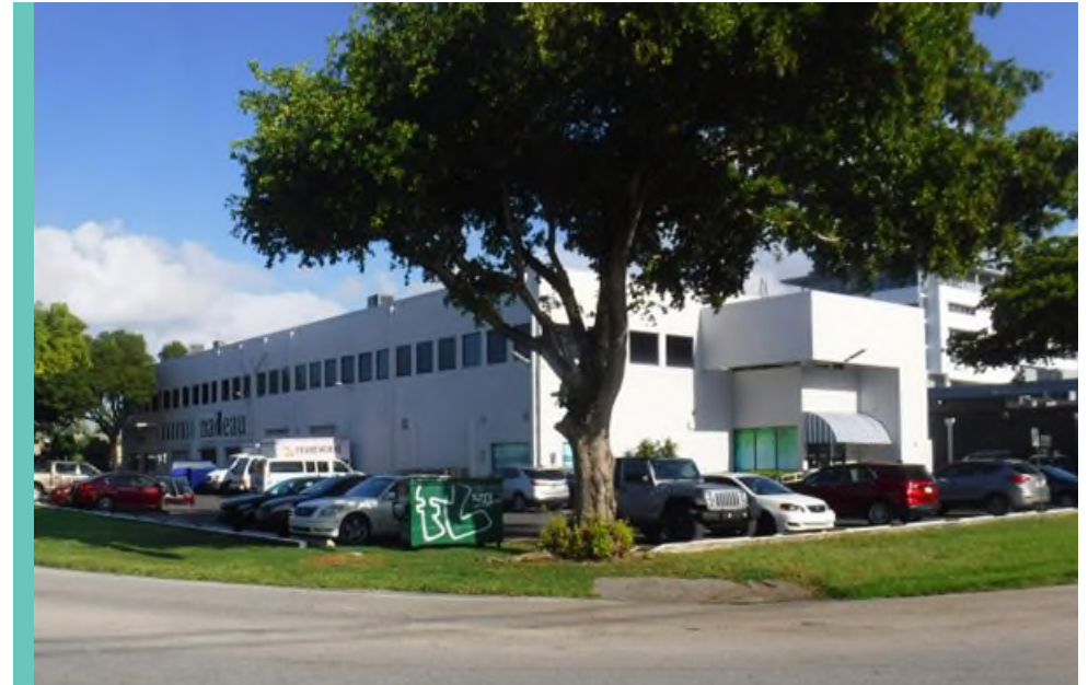
An International Style commercial building at 4180 SW 74th Court (Miami-Dade County), constructed in 1975 (8DA21573)
