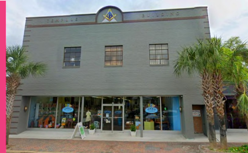
An example of alterations to a post-war (1960) commercial building at 130 SE Brooks Street (Okaloosa County). Alterations include modern windows and entrance.
