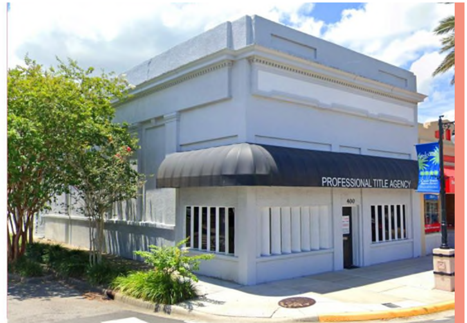
An example of alterations to a pre-war pre-war (1924) commercial building at 400 Canal Street (Volusia County). Alterations include modern windows, awnings, and entablature.
