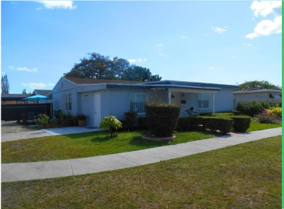
A structure with major alterations at 3401 SW 76th Avenue (Miami-Dade County), constructed in 1952. Alterations: new windows, enclosed car to make a second entrance
