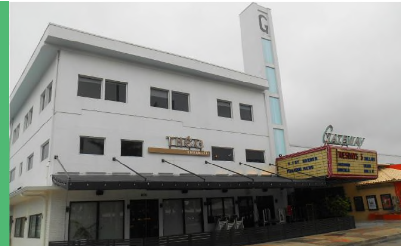
An example of alterations to a post-war (1950) commercial building at 41 NE 19th Avenue (Broward County). Alterations include the addition of a third story, modern windows and entrance. Alterations to the original vertical sign.
