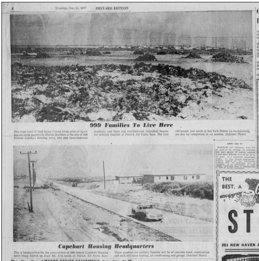
Figure 5: Newspaper article describing the Capehart Housing being constructed at Patrick Air Force Base (Brevard County) (Courtesy of The Orlando Sentinel, November 21, 1957)
