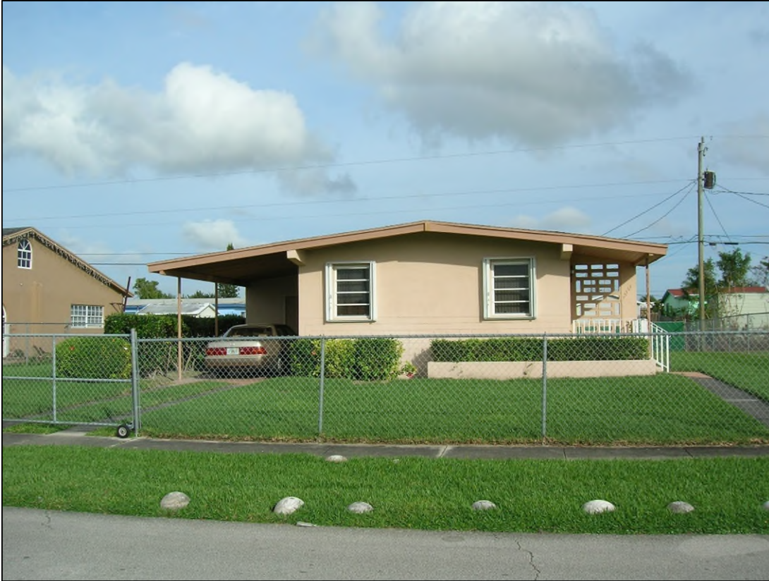
Figure 18: Representative Photo of House Type 3: 13721 Jackson Street, Facing Northwest
