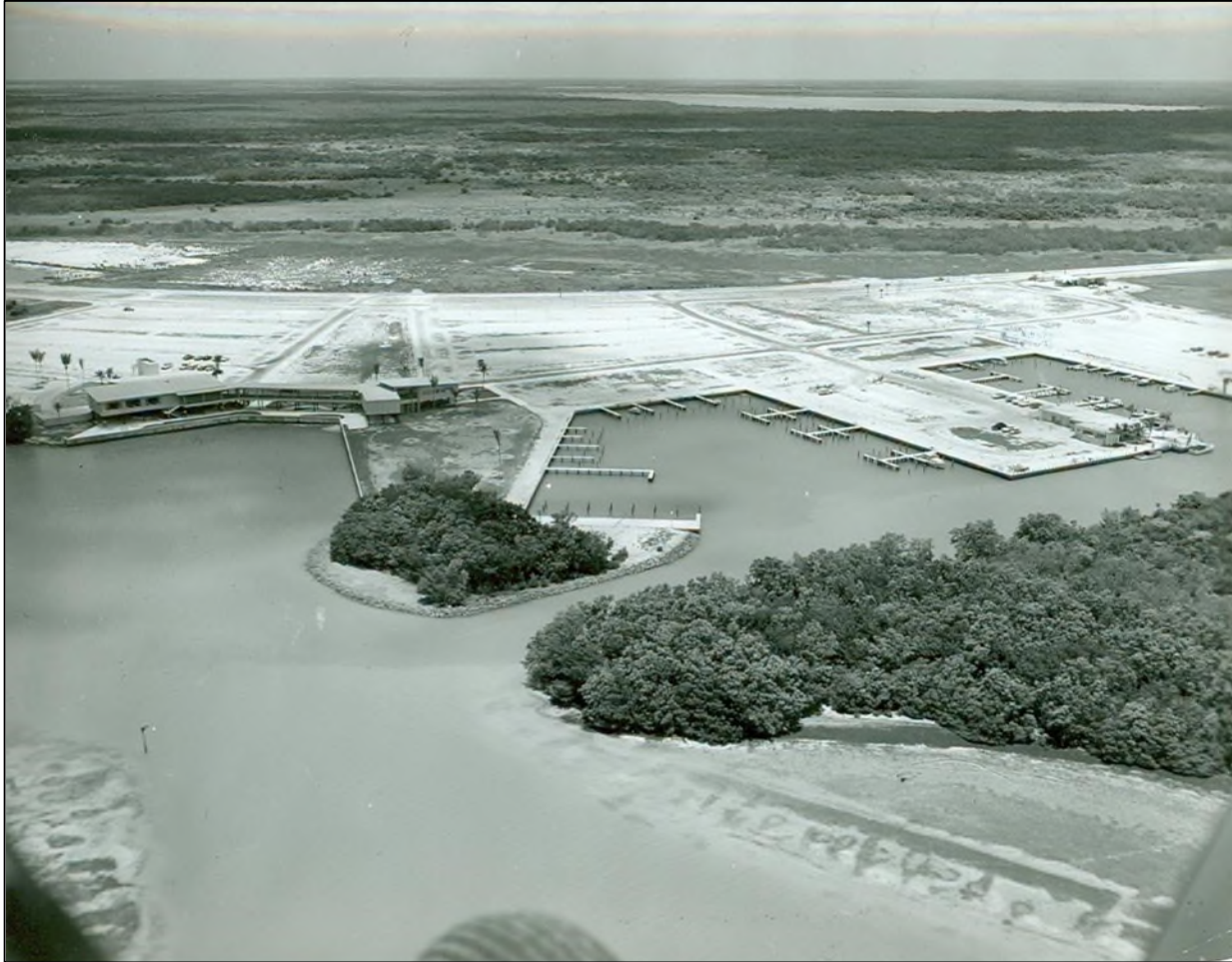
Figure 53: Aerial Photograph of the Flamingo Visitor Center and Marina under construction, ca. 1963, at the Everglades National Park. This complex was constructed as part of the Mission 66 efforts undertaken by the National Park Service (Courtesy of NPS-Mission 66)
