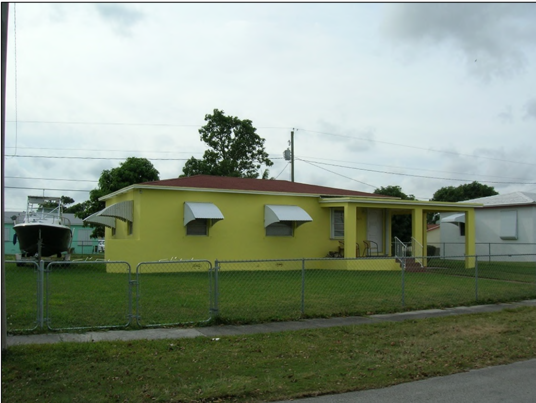
Figure 17: Representative Photo of House Type 2: 14560 Fillmore Street, Facing West
