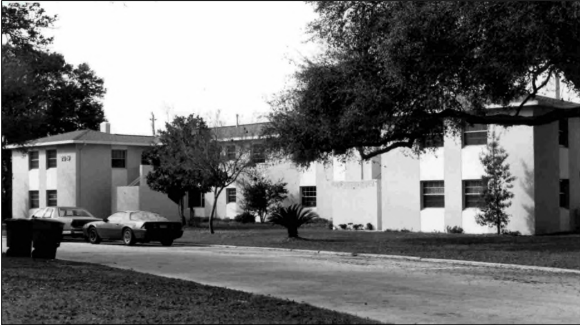
Figure 6: Example of a Wherry Multi-Family Housing Structure on McDill Air Force Base (Hillsborough County) (Florida Master Site File 8HI7851), facing Southwest
