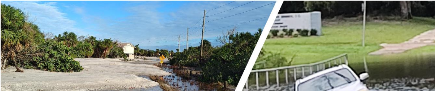
Damage from Hurricanes Debby, Helene & Milton, District 1, 2, & 7
