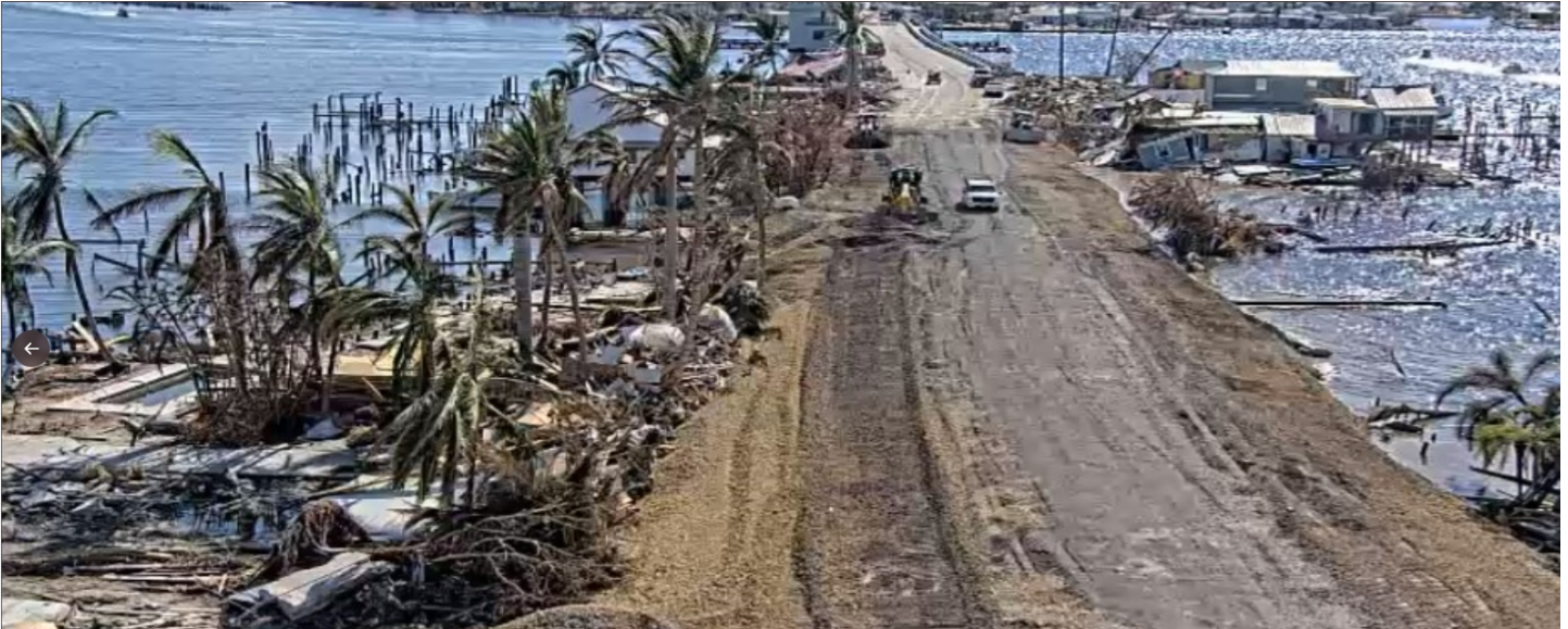
Bridge Repairs at Pine Island from Hurricane Ian, District 1
