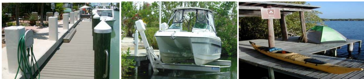
Figure 11. Pile-supported Structures. Example of a marginal dock on the left, boatlift with I-beam in the middle, and a chickee on the right. (The left and middle photos were provided by the Florida Marine Contractors Association and right photo from www.cnn.com ).
