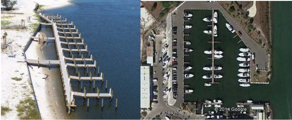
Figure 12. Sample Marina Images. The left image shows an example of an open water marina (provided by the Florida Marine Contractors Association), while the right image shows an example of marina contained within an upland cut basin (©2014 Google).
