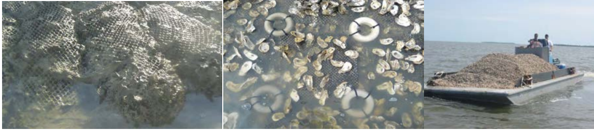
Figure 18. Oyster reefs. The left image shows oyster bags, the middle is an oyster mat, and the right is a barge filled with loose oyster cultch. All 3 images are from the Charlotte Harbor Habitat Restoration Plan (Boswell et al. 2012).
