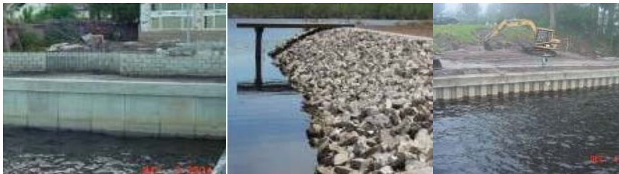
Figure 9. Example images of shoreline armoring and stabilization. The left image is a concrete slab seawall, the middle is a riprap shoreline, and the right is a vinyl seawall. (Images provided by the Florida Marine Contractors Association in 2014).
