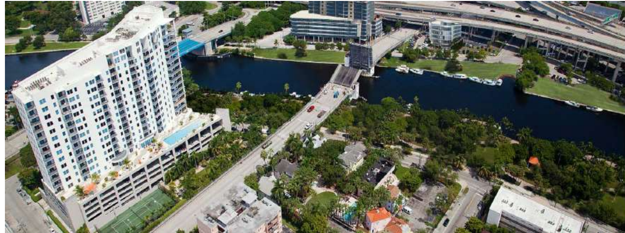
First Street Bridge before construction
