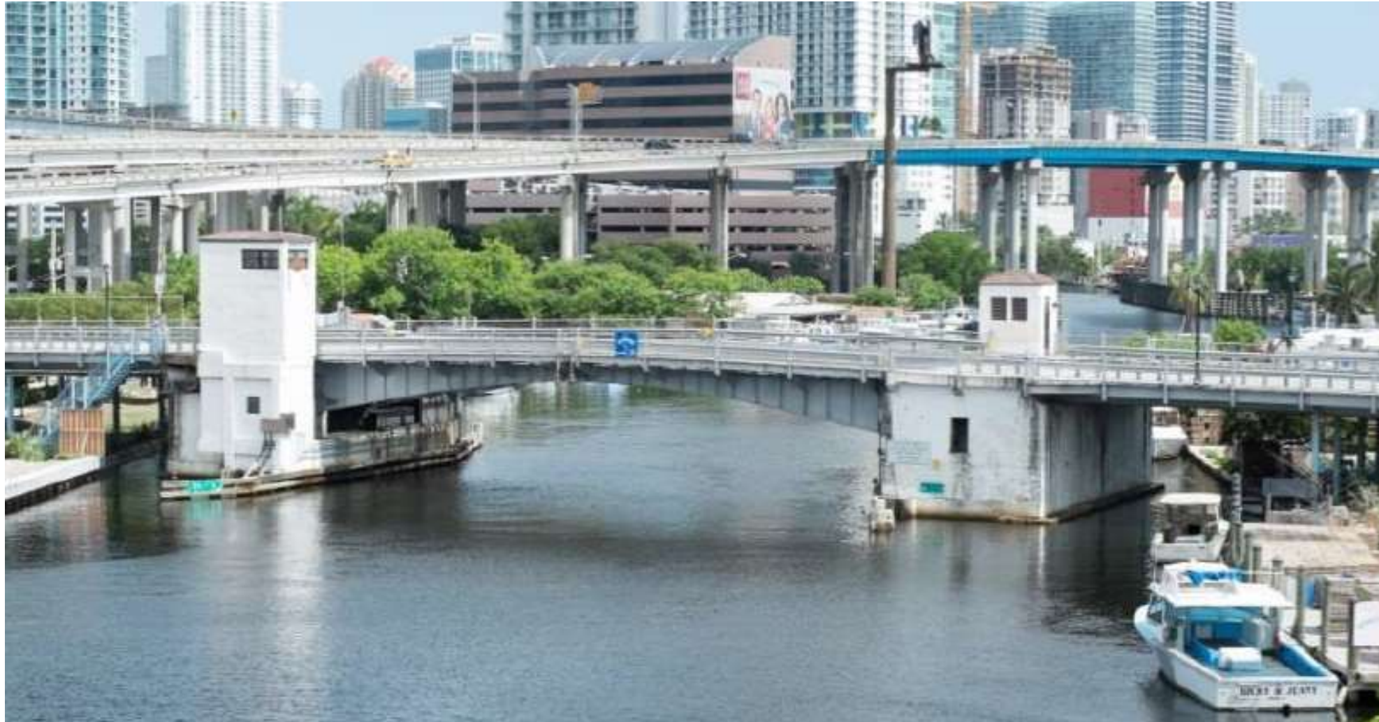
First Street Bridge before construction
