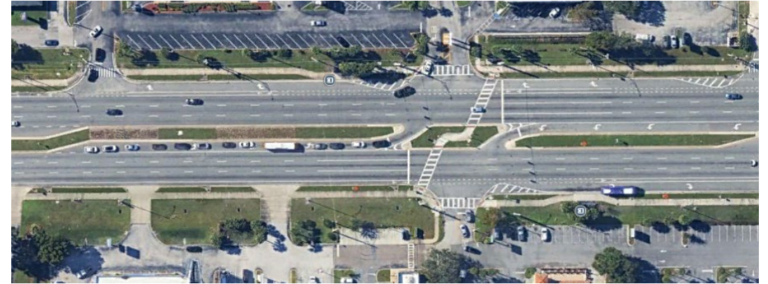
Signalized RCUT – Orlando, FL
