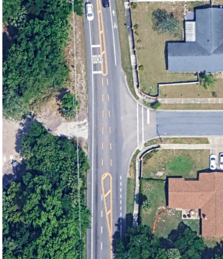
Minor Road Stop Control – Oviedo, FL
