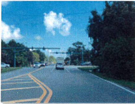
1 South End at Begin Project.JPG
