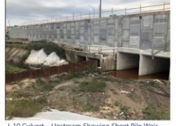
I-10 Culvert – Upstream Showing Sheet Pile Weir
