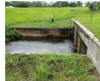
c) Concrete weir box at upstream end of culverts
