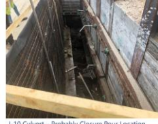
I-10 Culvert – Probably Closure Pour Location
