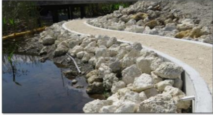
Figure 11 Example of a Crossing Retrofit: A dry shelf with a pathway to transition between end of dry shelf and natural ground at Harold Strand, I-75 Alligator Alley, Collier County, D1 (FPID 444008-3). PVC pipe in right foreground is a drainage feature for the walking surface.
