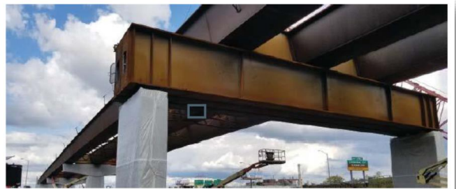
Figure 2.3-2: Non-integral, Stacked Connection
