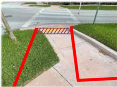
Curb Ramp Alignment Detectable Warning Surface
