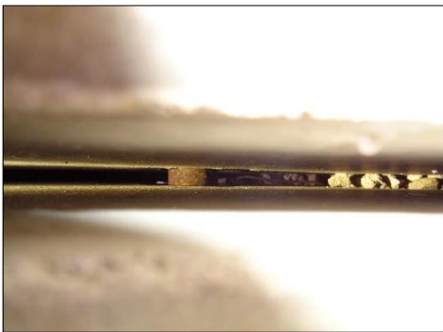
PHOTO 3 – ELEMENT 8099 (W/O) TYPICAL VIEW OF TRANSVERSE POST TENSIONING BARS WITH SURFACE CORROSION
