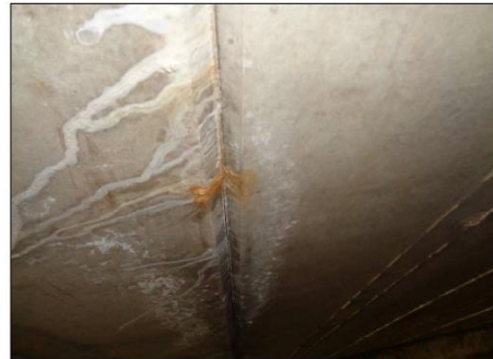
PHOTO 6 – ELEMENT 8099 TYPICAL VIEW OF EFFLORESCENCE AND CORROSION BLEEDOUT EMITTING FROM LONGITUDINAL JOINT BETWEEN SLAB UNITS
