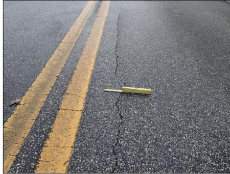
PHOTO 10 – ELEMENT 8099/510 TYPICAL VIEW OF UP TO WIDE SIZE LONGITUDINAL CRACKS IN ASPHALT SURFACE OVER SLAB UNIT JOINTS AT RANDOM LOCATIONS
