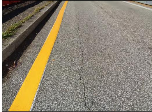
PHOTO 10 – ELEMENT 8099/510 VIEW OF UP TO MODERATE SIZE LONGITUDINAL CRACKS IN ASPHALT WEARING SURFACE
