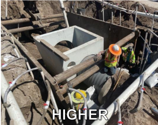
0430-17A-BCC – Pipe Culvert Optional Material – Excavation or Trenching
