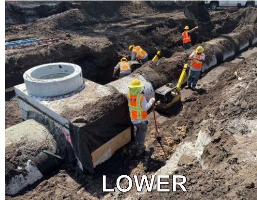
0430-17A-BCC – Pipe Culvert Optional Material – Excavation or Trenching
