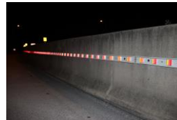
Delineators along exit ramps
