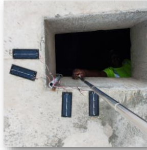
Panels mounted on the underside of bridge
