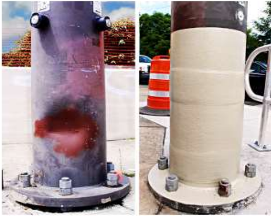
This utility pole (left) was damaged in a collision, but it was successfully repaired (right).
