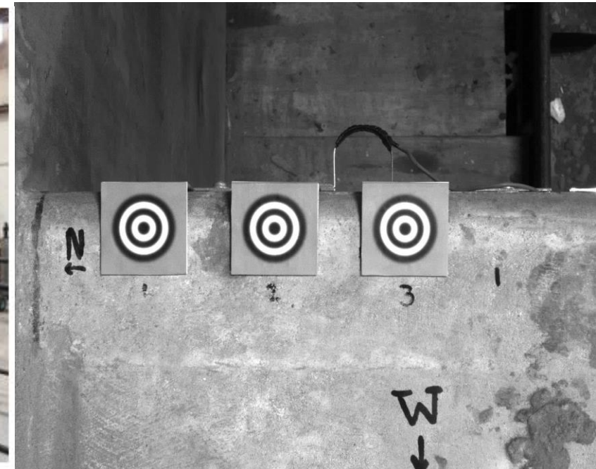
CRACK OPENING TRACKING BY IMETRUM CAMERA
