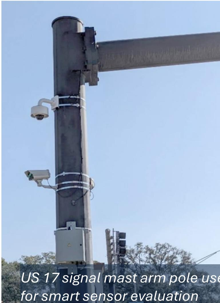
*US 17 signal mast arm pole used for smart sensor evaluation*
