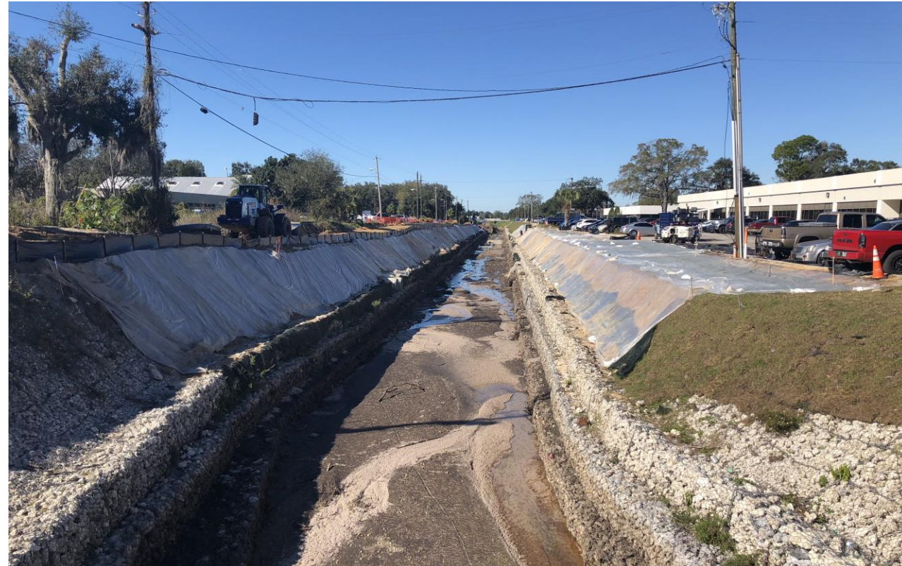
Temporary Construction Easement – Removed Trees to Prevent Property Damage
