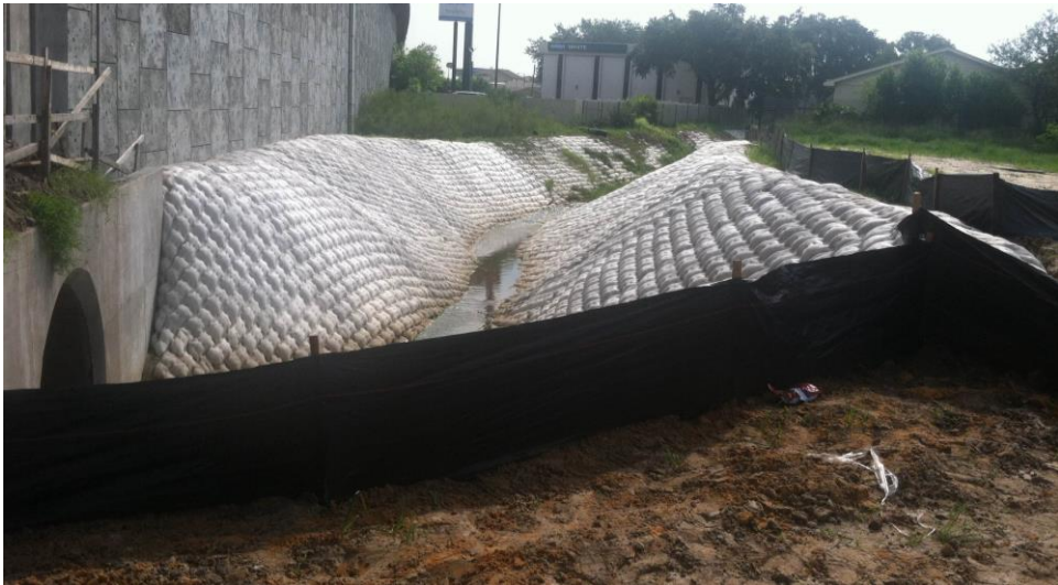
Construction of Henry Canal
