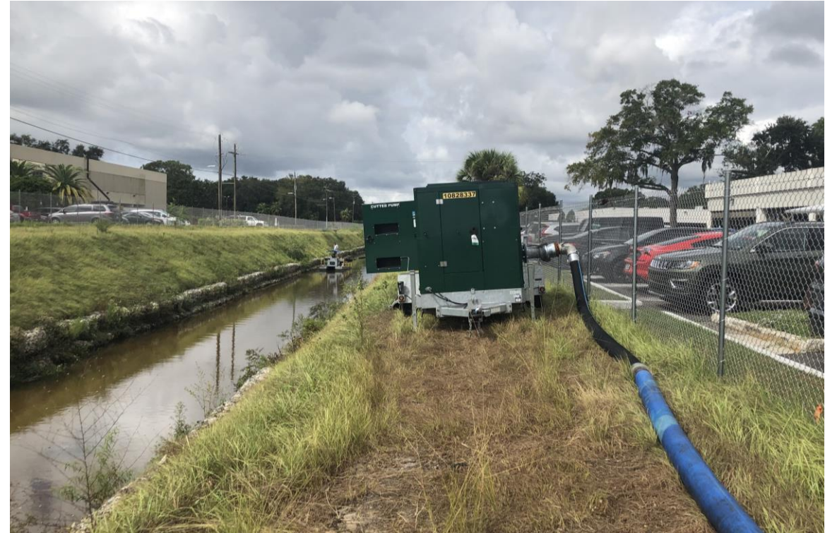
Water Bypassing Plan – Used pumps redirect water from work zone.
