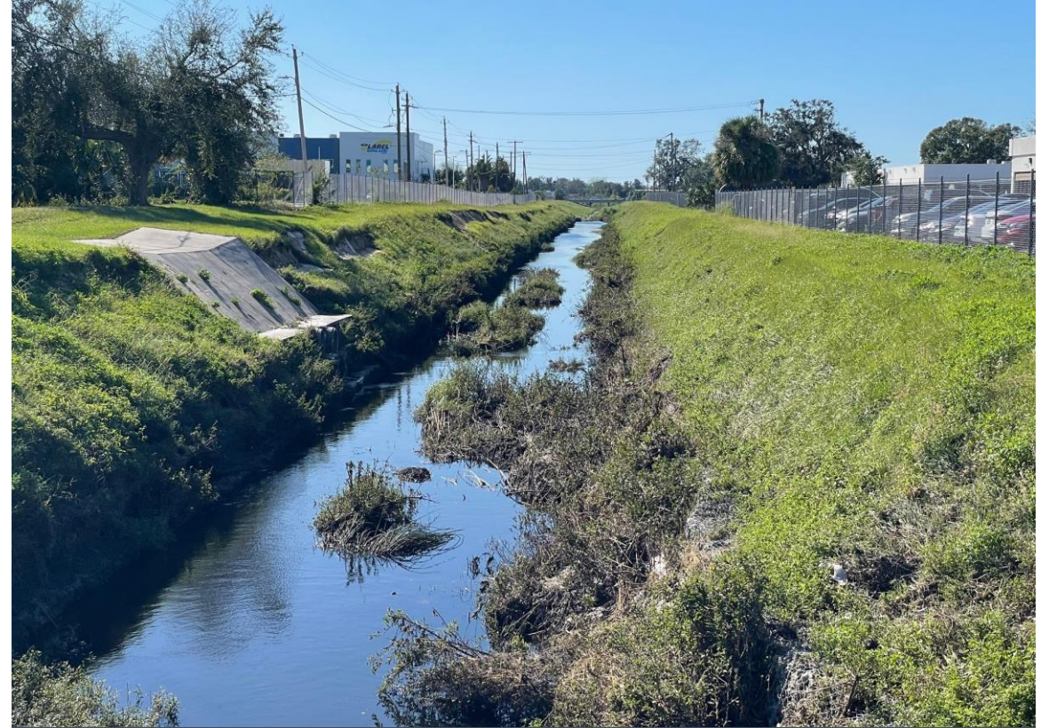
Post Hurricane Milton Henry Canal Segment 3 (October 2024)
