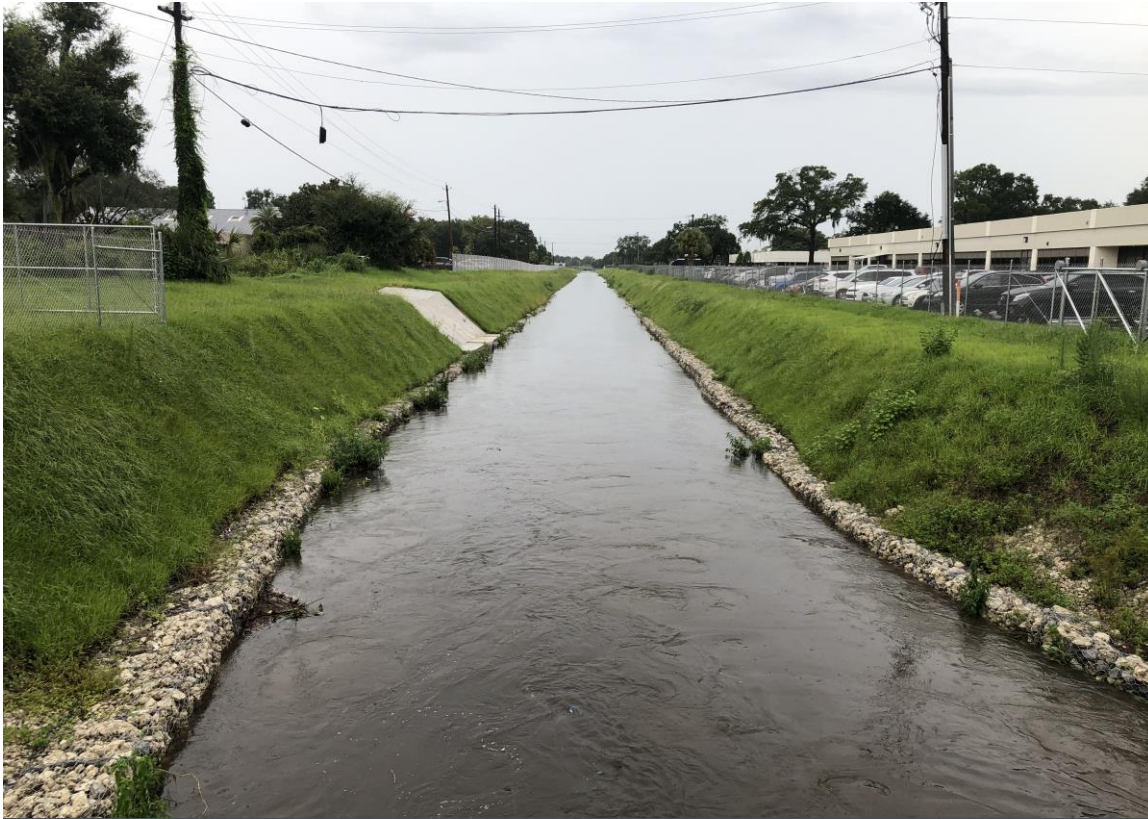
Construction Complete: Henry Canal Segment 3 (July 2019)
