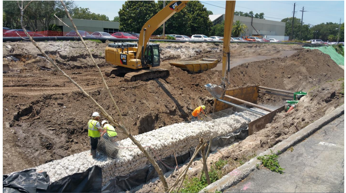
Construction of Gabion Baskets
