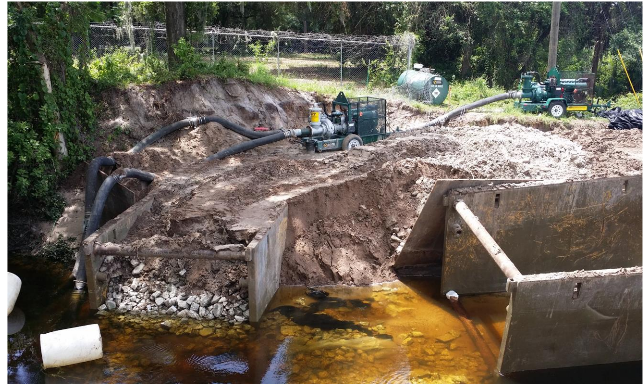
Temporary Drainage – Trench Box
