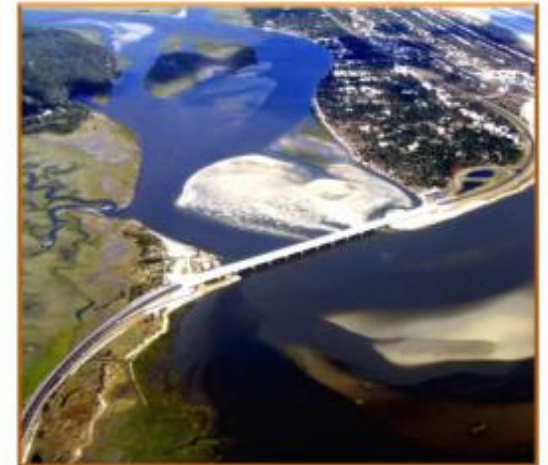
Fort George/Talbot Island Bridge, FL
