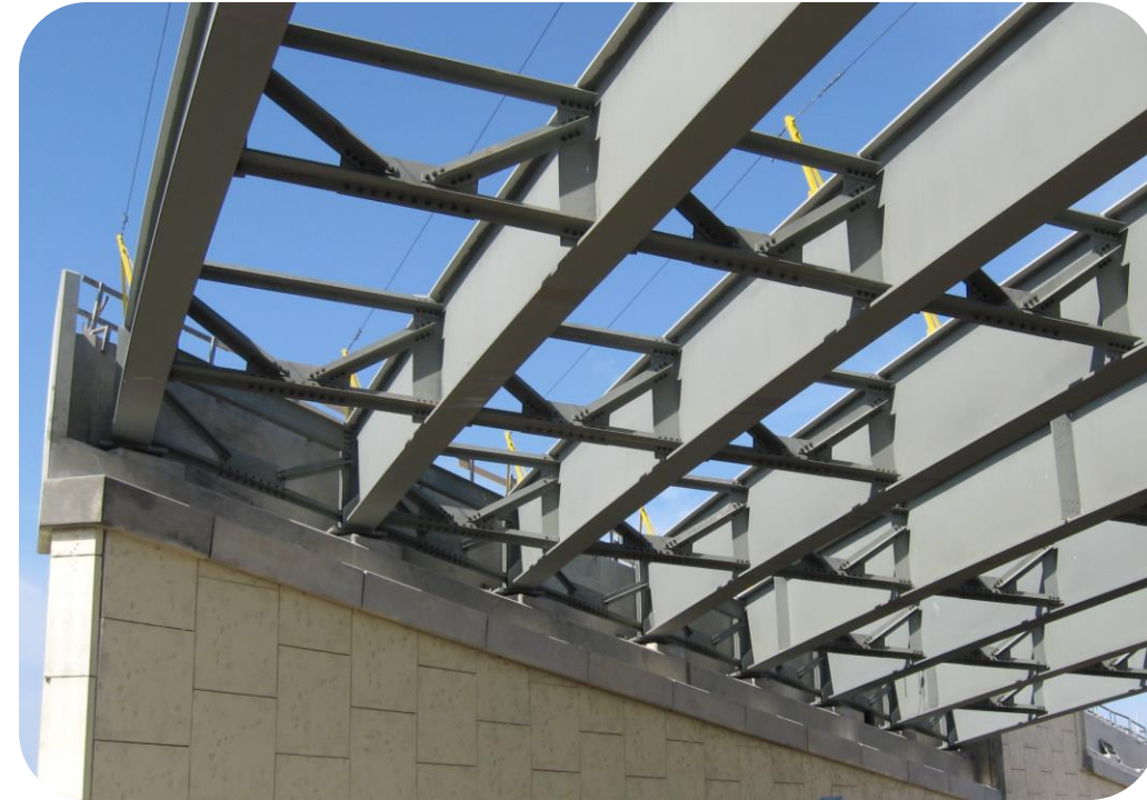
Straight Steel I-Girder (SSI-G)
