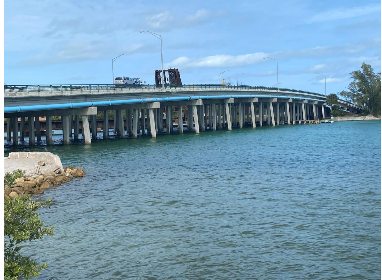
SR 811 (Alt. A1A) Bridge Rehabilitation
