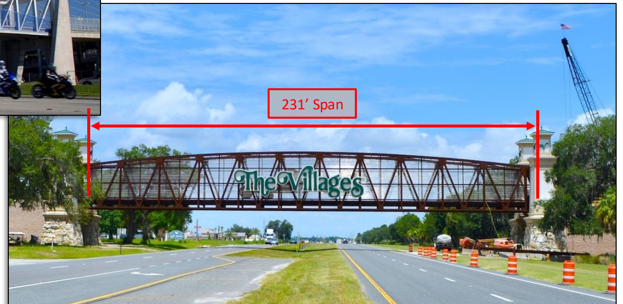
The Villages Water Lily Bridge over the Turnpike
