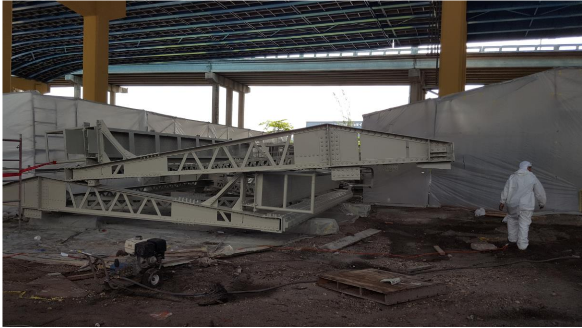
Contamination remediation & repainting
