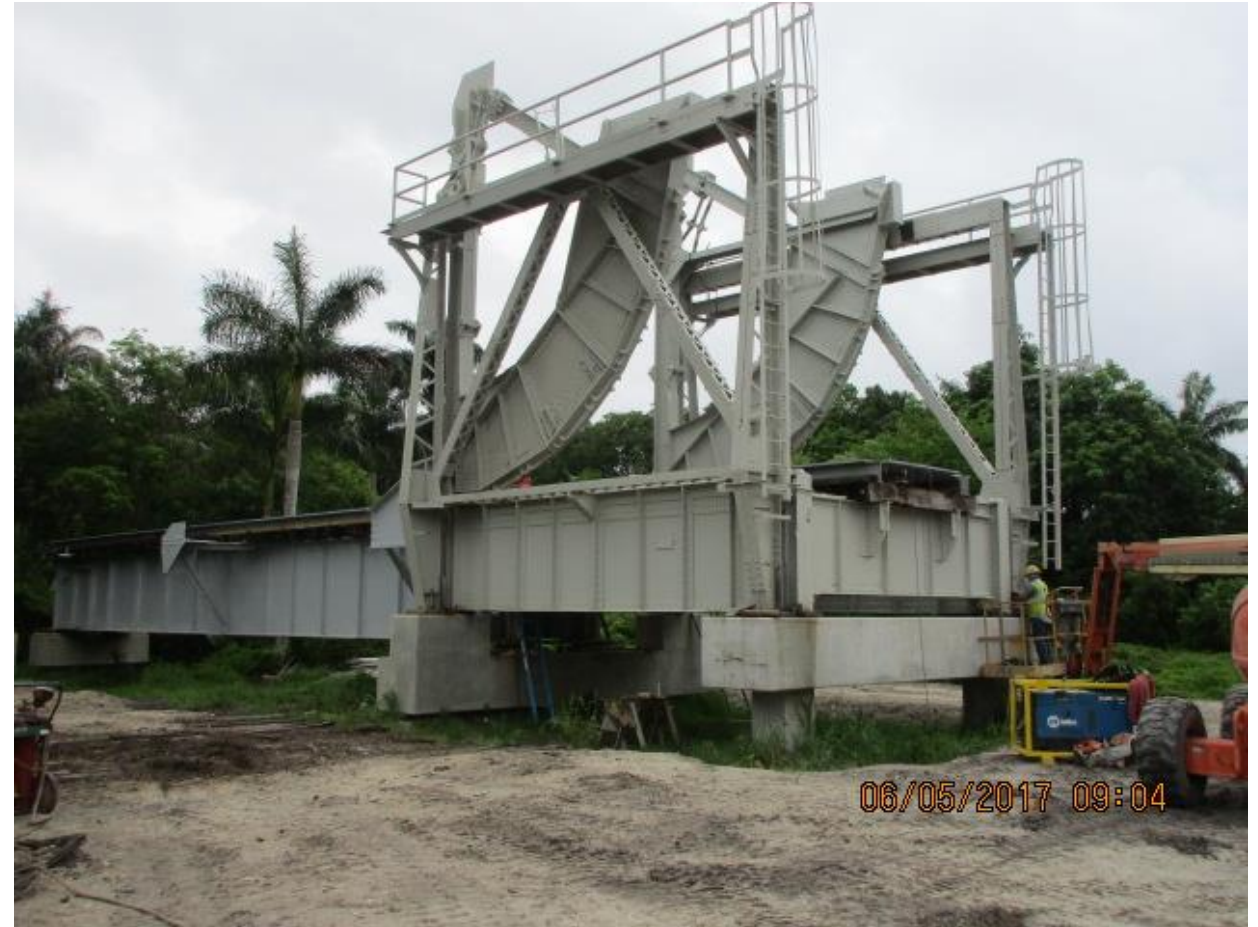
Reassembly on the site
