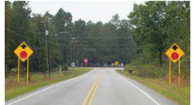
Source: South Carolina DOT
