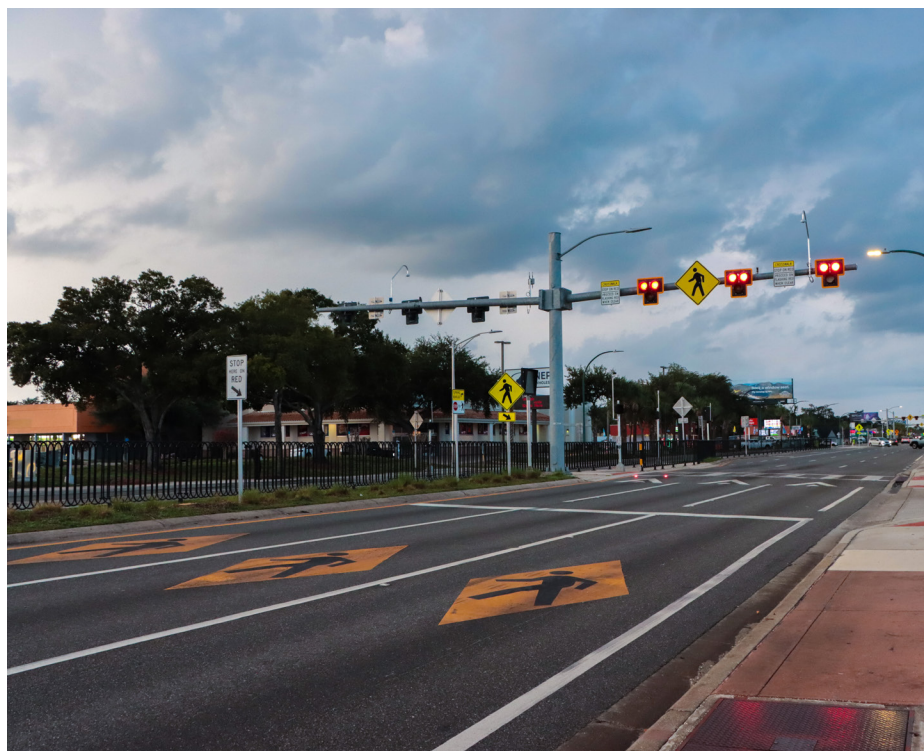
In-lane pedestrian warning markings
