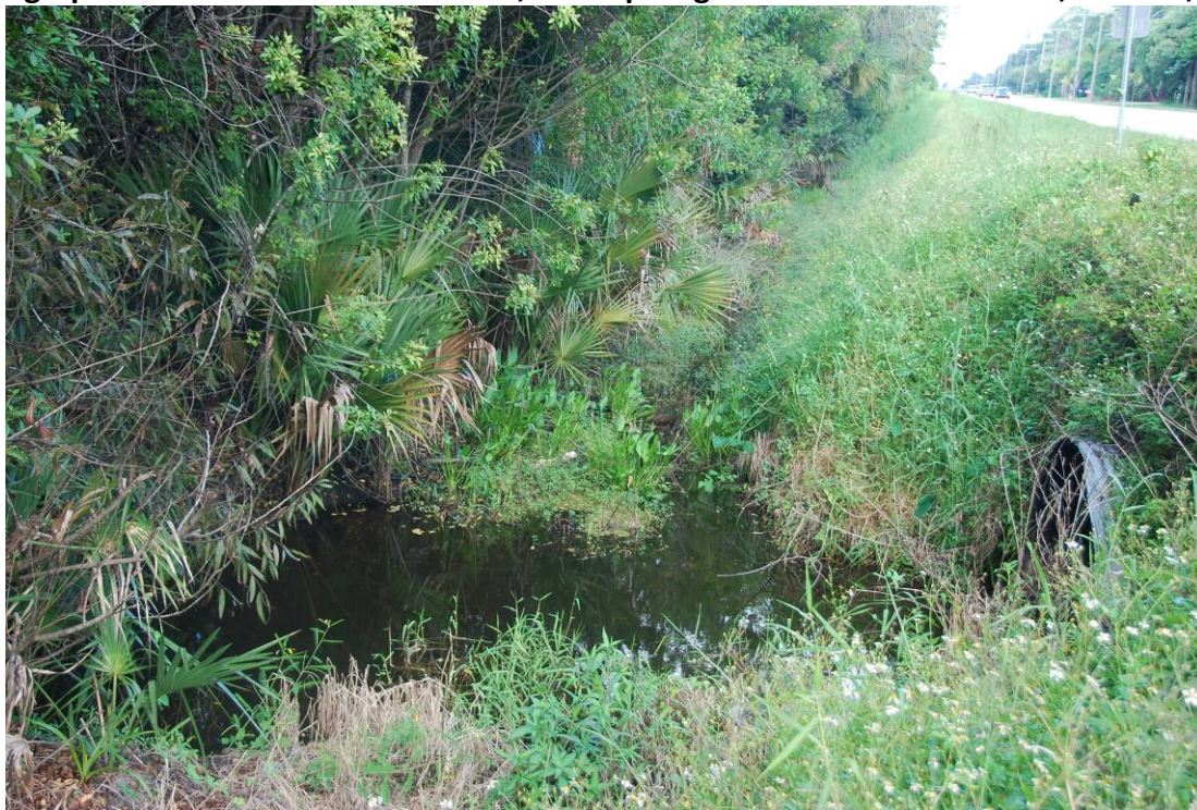
6 7 Photograph 8-2 Culvert Outfall, AA7, south prong Saint Sebastian River, September 28, 2016
