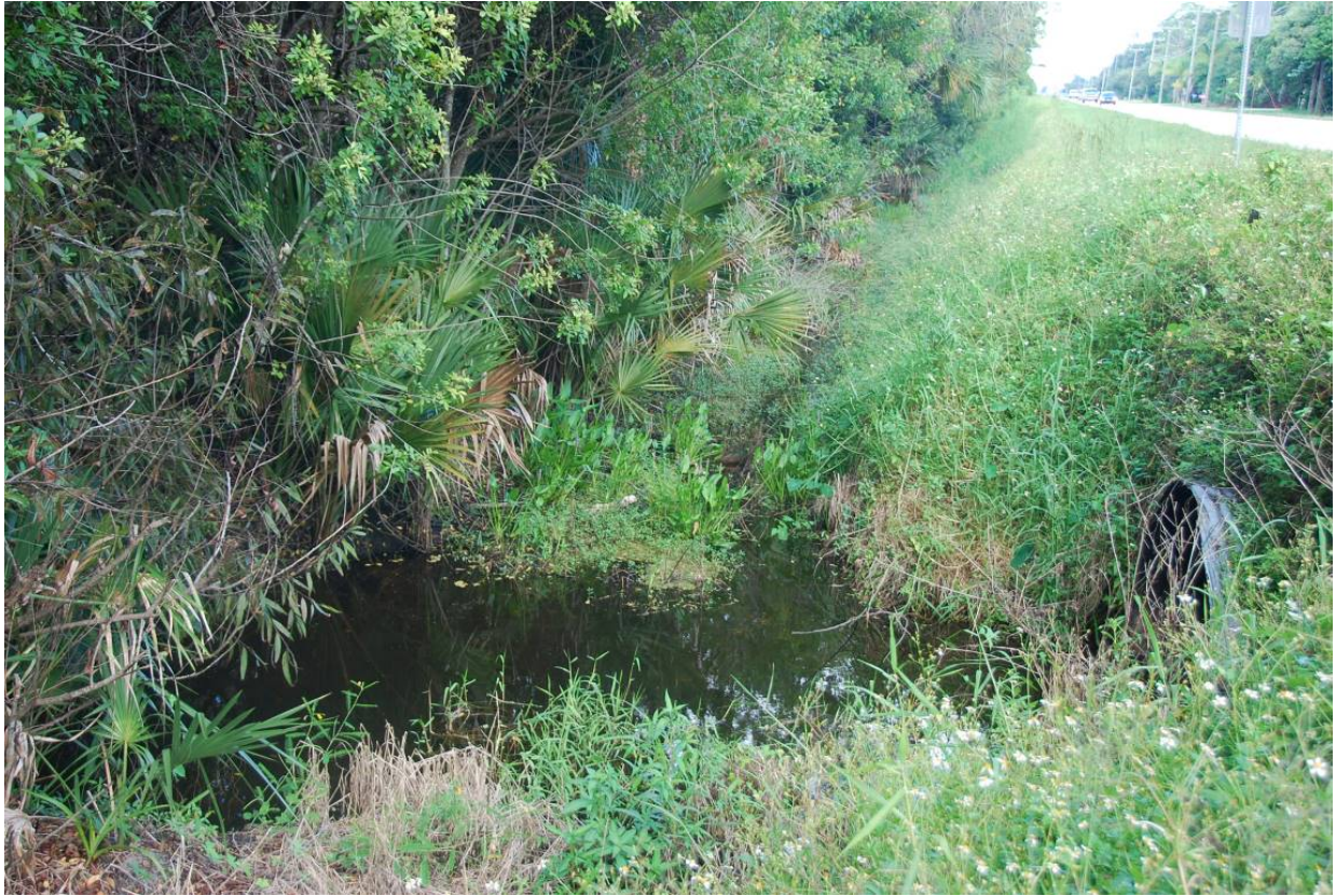
Photograph 1 South Prong of St. Sebastian River Culvert at C.R. 510, Facing East
