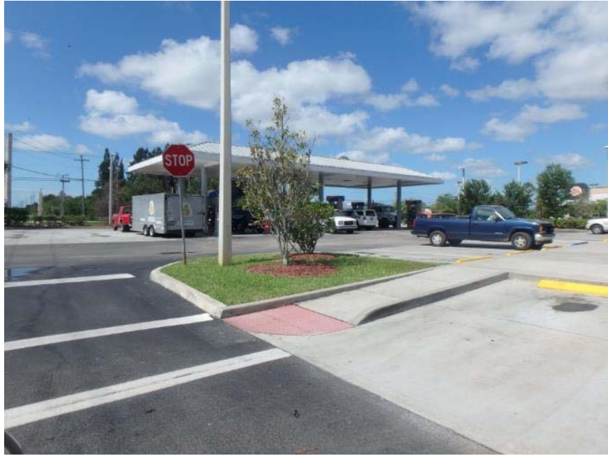
Photo 3: View of interior of site facing northeast
