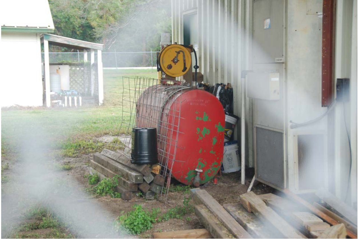
Photo 8: Fuel tank at Ryall Groves Inc., facing north
