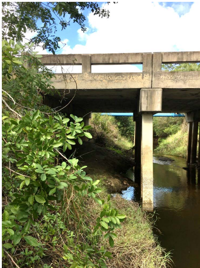
Canal D Bridge Foundation
