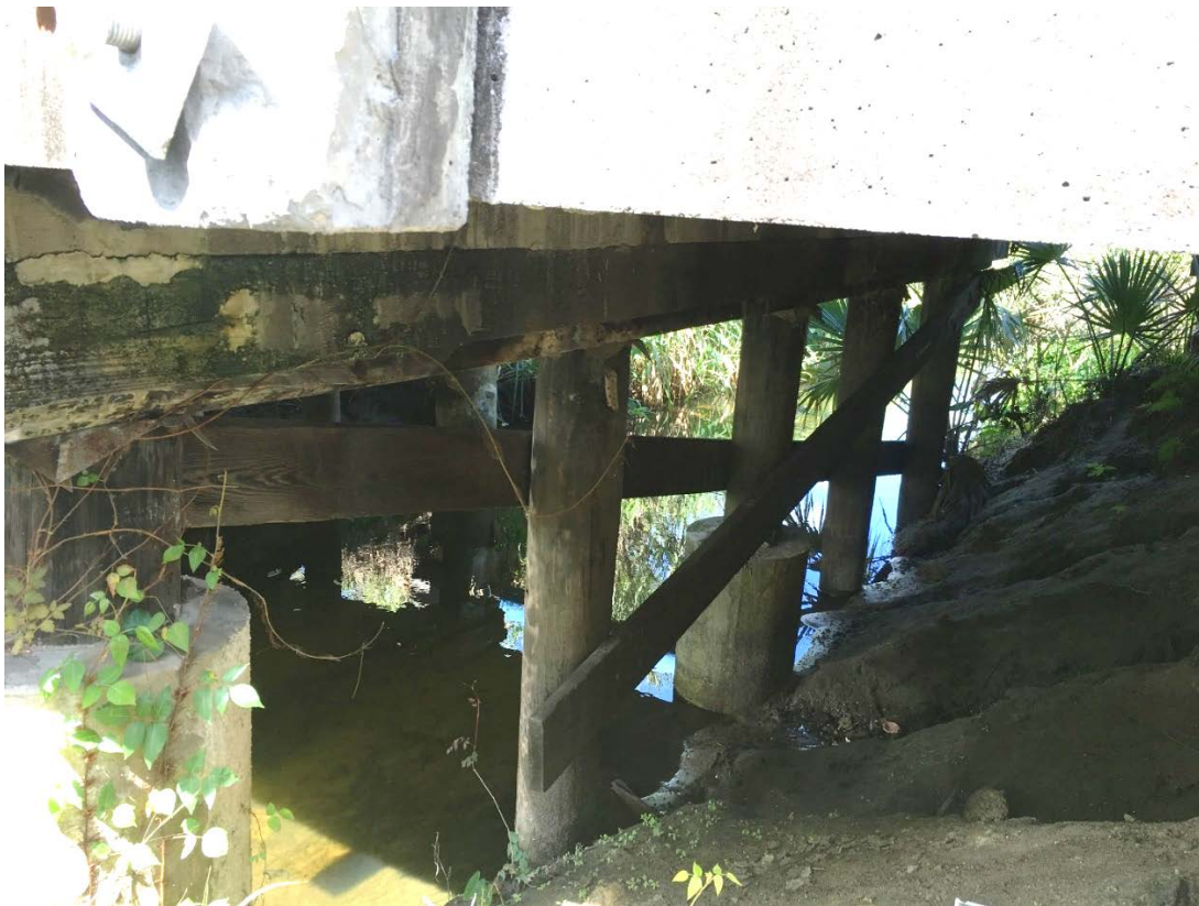
Canal L Bridge Foundations
