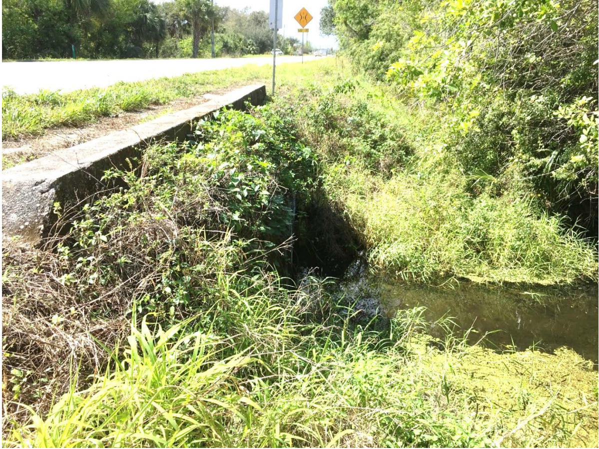
Canal Slough Downstream
