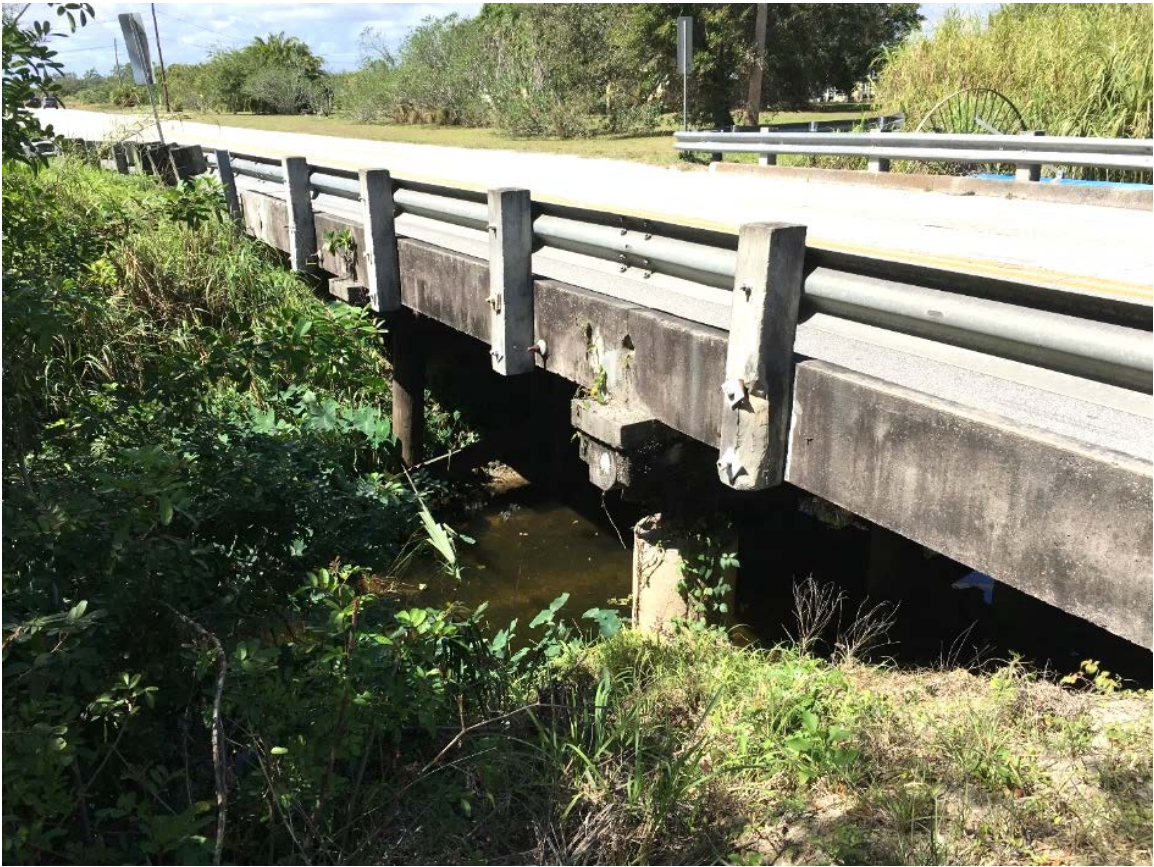
Canal L Bridge Piers
