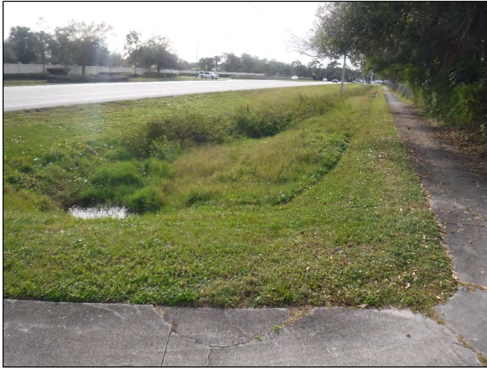
Figure 10: North Side of Cove Road Illustrating a Wet Ditch, a Spoil Berm with a Fiber Optic Cable and Sidewalk, facing West-Southwest
