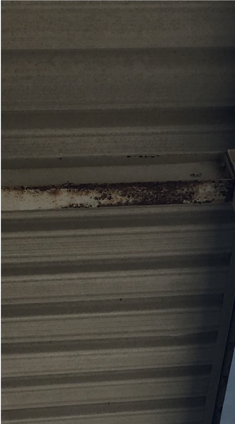
All mill scale rust to be removed prior to Primer application
