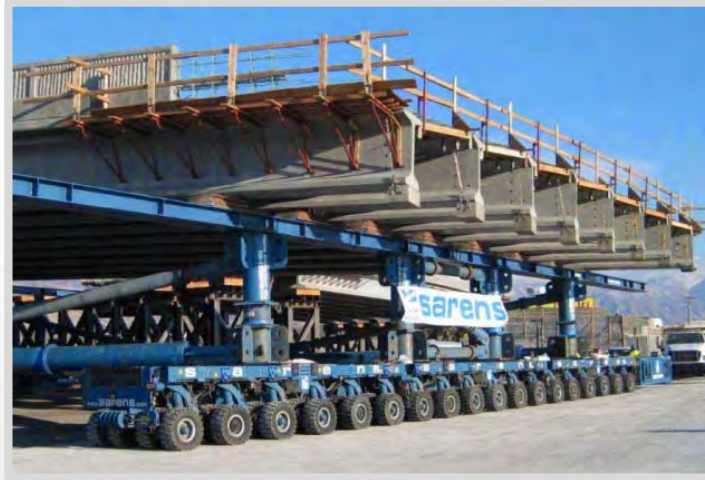
SPMT Removal/Installation
