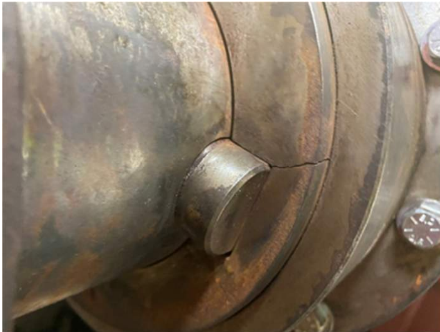
Photo 2: Note “visible gap between hub and shaft and “opened” crack
