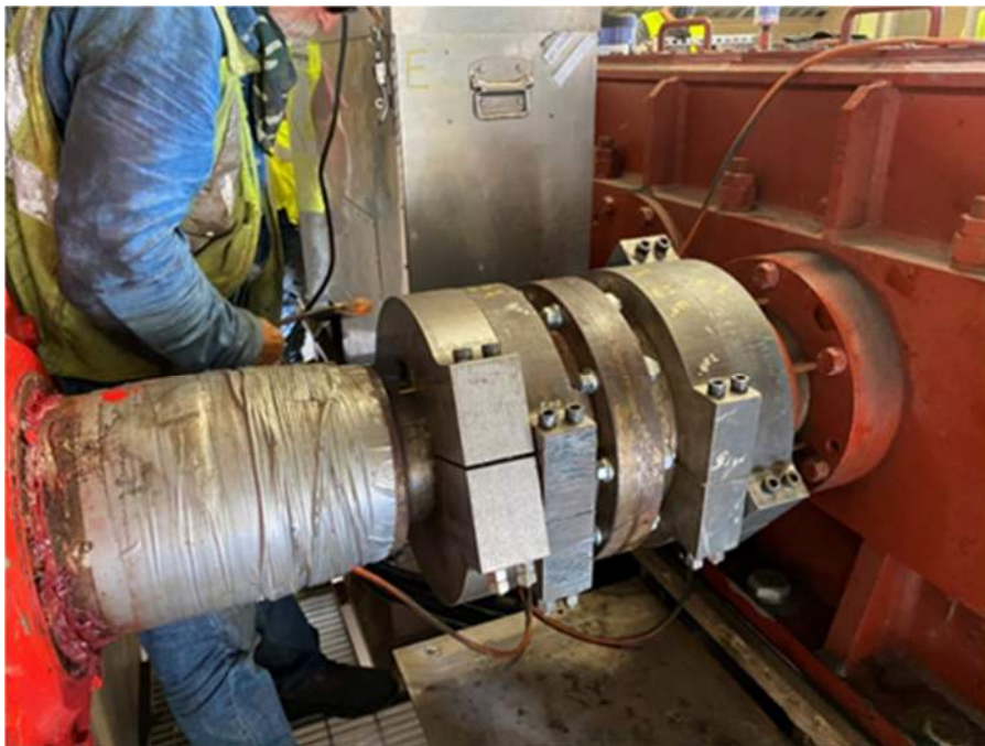
Photo 8: East coupling clamped with steel bands
