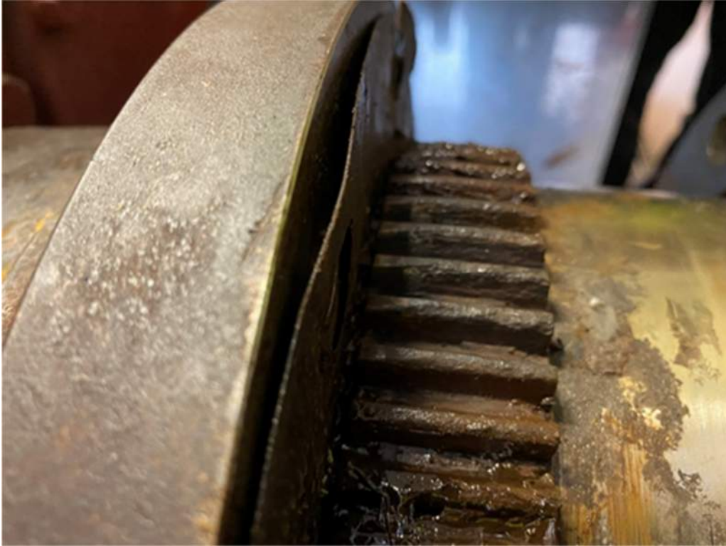
Photo 7: Corroded and worn west reducer hub gear teeth
