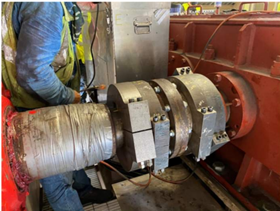
Photo 8: East coupling clamped with steel bands
