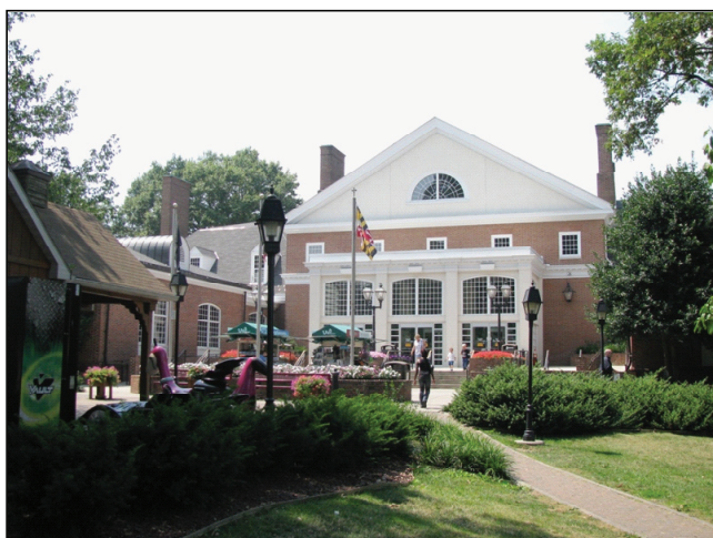
Exterior facade of Maryland House
