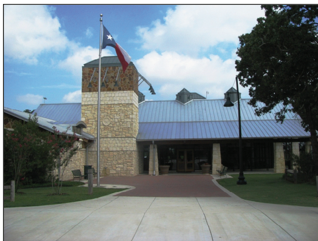
Regional vernacular architecture example
