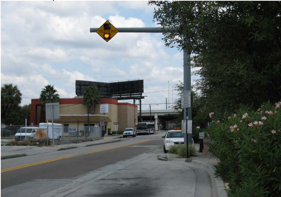
Figure 51 Yield-to-Bus Roadway Flashing Beacons
