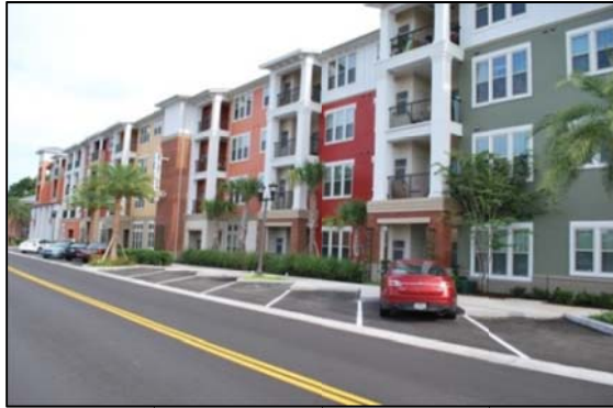
Figure 6-2: Station House Apartments
