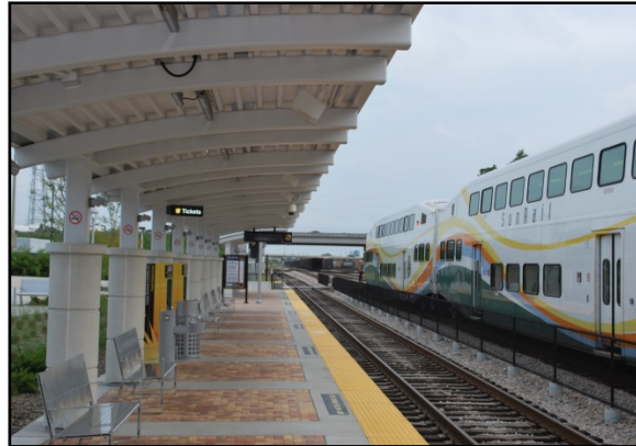
Figure 11-1: Sand Lake Road SunRail Station
