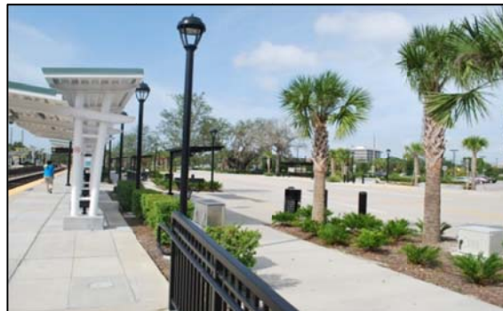
Figure 8-1: Altamonte Springs SunRail Station
