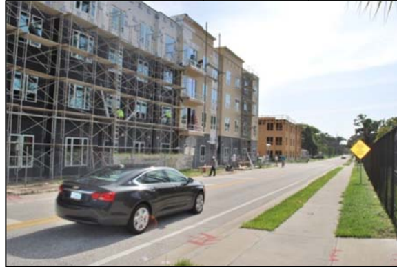
Figure 7-2: Weston Park Under Construction
