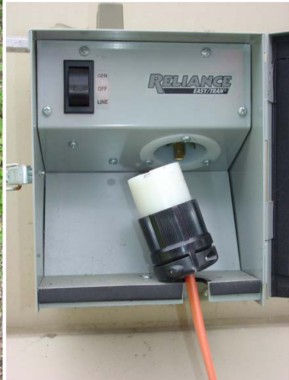
Generator Cable Twist Lock Connector can be secured to transfer switch with pad lock.
